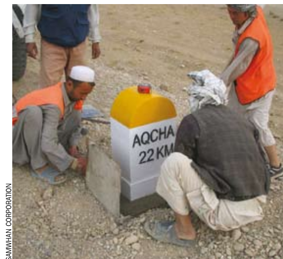
FINAL TOUCHES Road markers are installed along the rehabilitated road from Balkh to Andkhoy.
