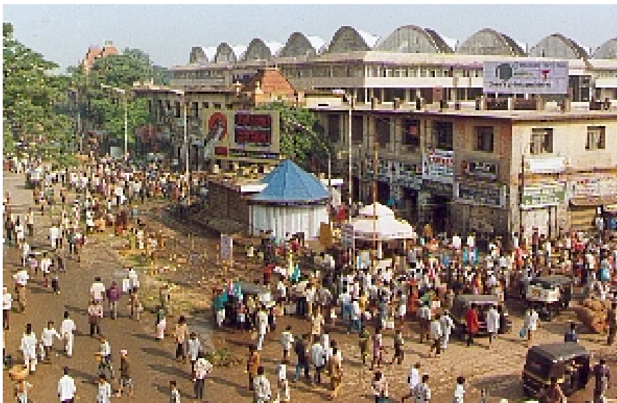
New multistoried markets like the Shri Khrisnarajendra City Market are being constructed
