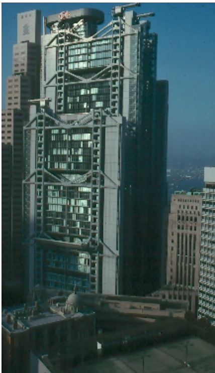
Headquarters of the Hong Kong and Shanghai Bank
