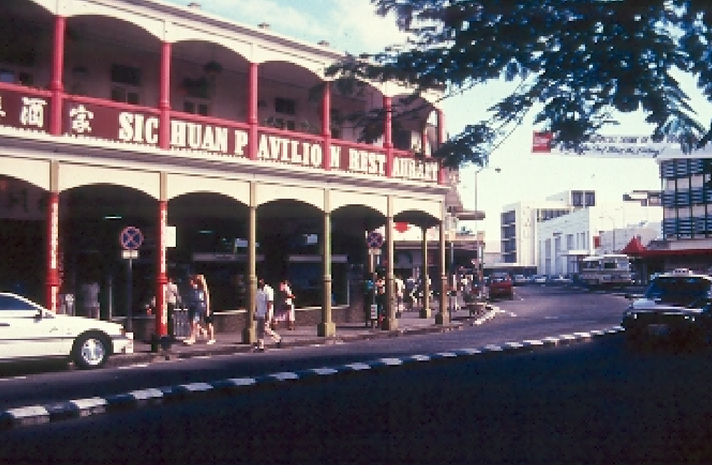
The city retains an old building at downtown area
