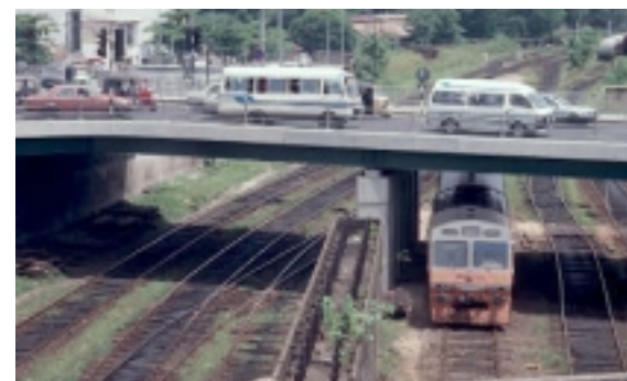
The government implements several rail and road projects to improve accessibility
