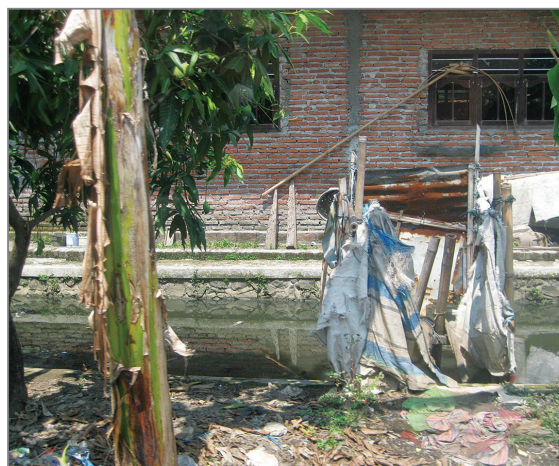
Informal sanitation. Overhung or hanging latrines, such as this one in Pekalongan, Indonesia, are suspended above water bodies; they are unhygienic and pollute rivers, canals, and the sea (photo by Isabel Blackett).
