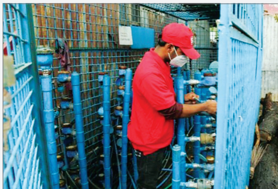
Asset protection. Shobar Jonno Pani protects clusters of water meters in locked cages in Bangladesh (photo by Shobar Jonno Pani).
