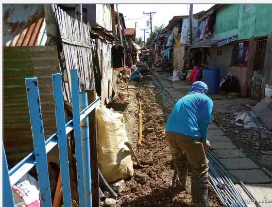
Water connection. Laying of pipes to clusters in Guizo community (photo by Tubig Pag-Asa, Inc.).
