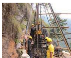
Core drilling at Tanahu HEP
