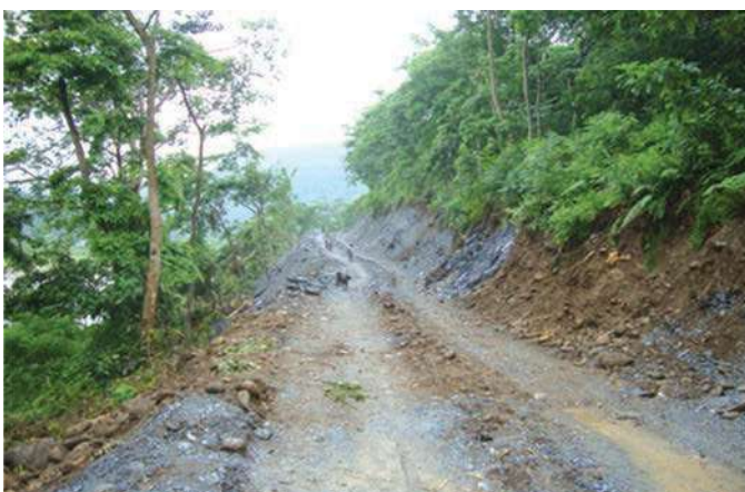
Under construction access road to Powerhouse site.
