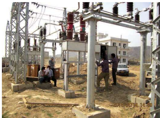
Construction Works of 33 kV S/S
