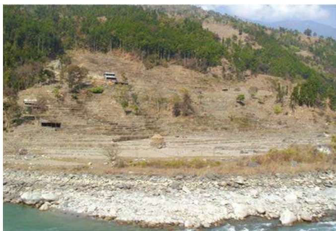
Proposed Powerhouse site
