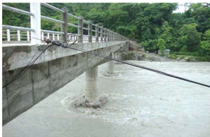
RCC Bridge over Seti River
