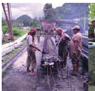
PSC Pole Production at Kotre Pole Plant
