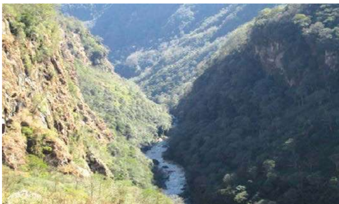
Upper Arun Headwork site
