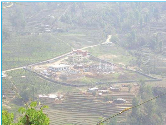
Godak (Ilam) 132/33 kV substation
