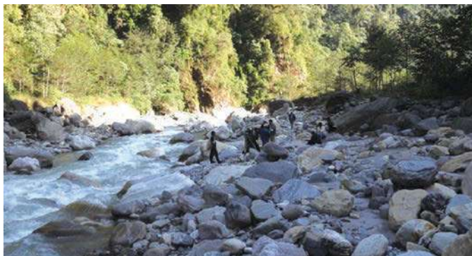
Upper Modi 'A' Headwork site
