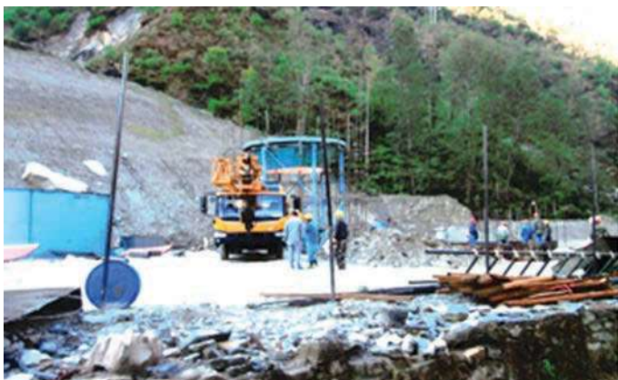
Batching Plant at Headworks
