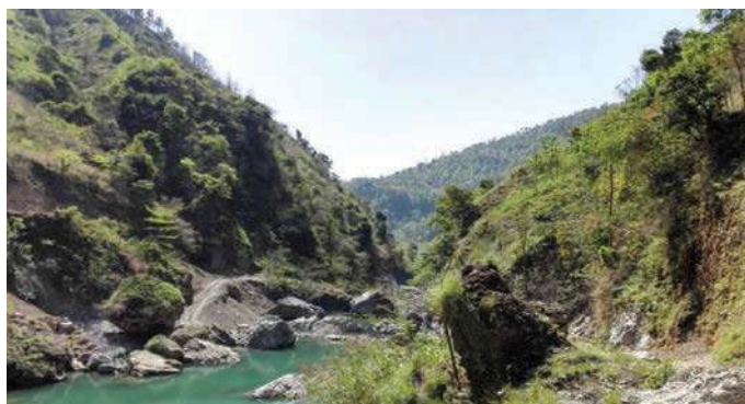
Andhikhola Dam Site
