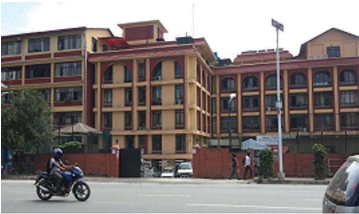
Intact NEA Central Office
