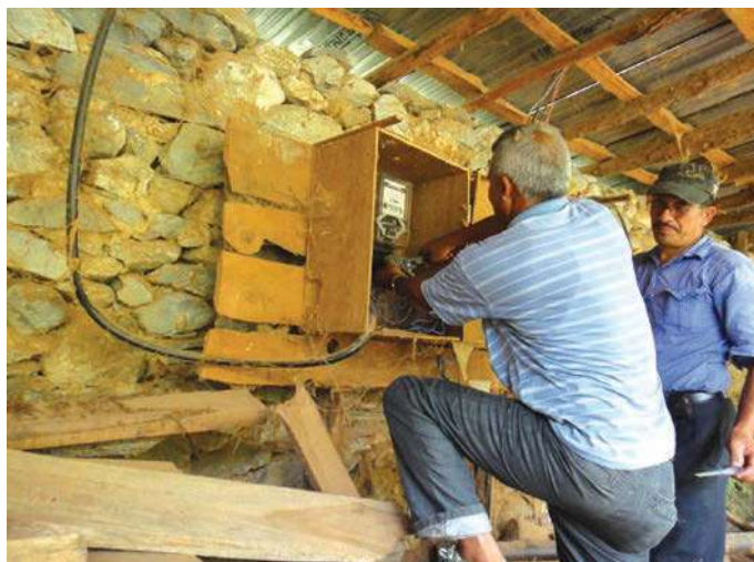
Meter resealing being done by NEA Employee
