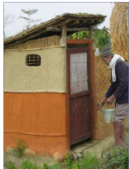
Permanent toilet with local materials above plinth level
