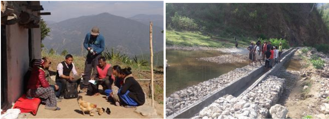
Picture 11. Sharing knowledge with community members and irrigation canal constructed
