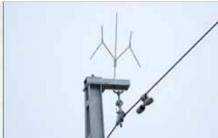
Wishbone Prevents Bird Landing on Wire
