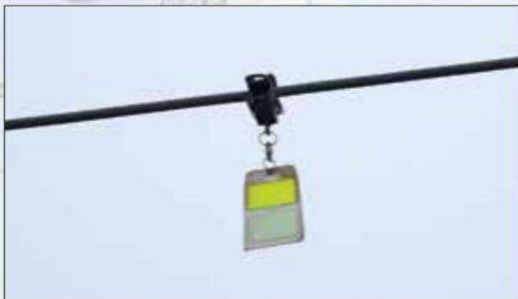
Bird Diverting Reflector
