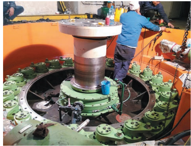
Assembly of Wicket Gate and Shaft of Turbine
