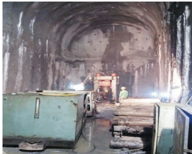
Drilling for Pilot Shaft in Penstock
