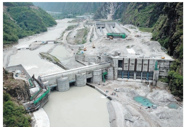
Headworks structure of UTKHEP.
