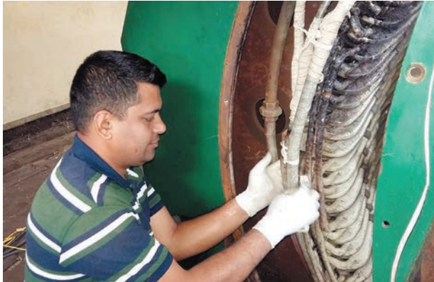
Stator Jumper Coil Repair (Unit # 1)
