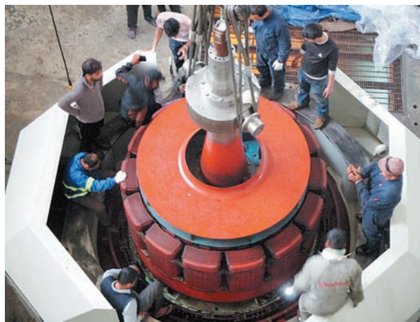
Rotor Being Removed for Overhauling (Unit #2)
