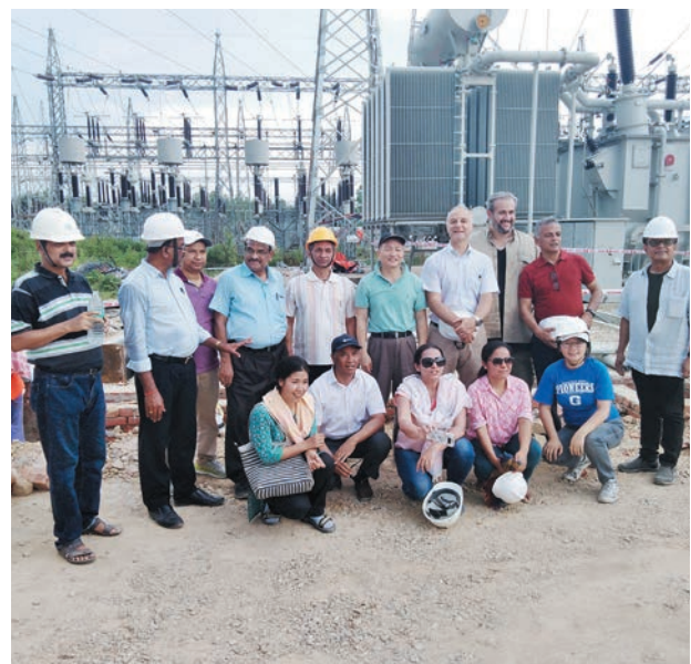
WB Team monitoring charging of 220/132 kV Transformer at Dhalkebar
