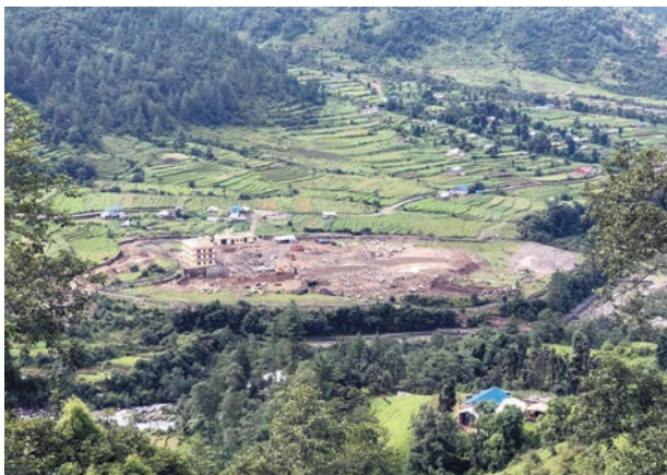
Underconstruction Garjyang 132 kV Substation
