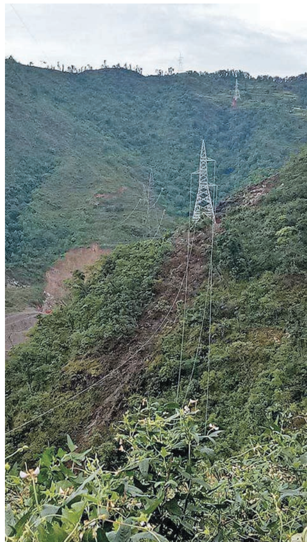
Re-routing of Marsyangdi-Kathmandu 132 kV Transmission Line
