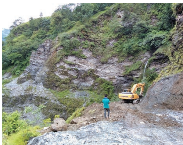
Access Road Construction on progress, Rahughat HEP
