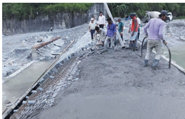
Seti Weir Construction Work
