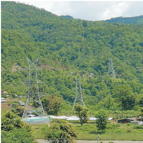
220 kV tower erected for Marsyangdi-Kathmandu T/L
