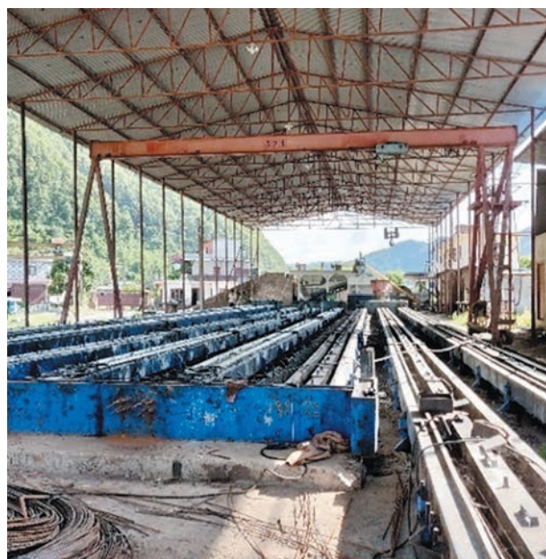
Pole Production at Kotre Pole Plant, Tanahu
