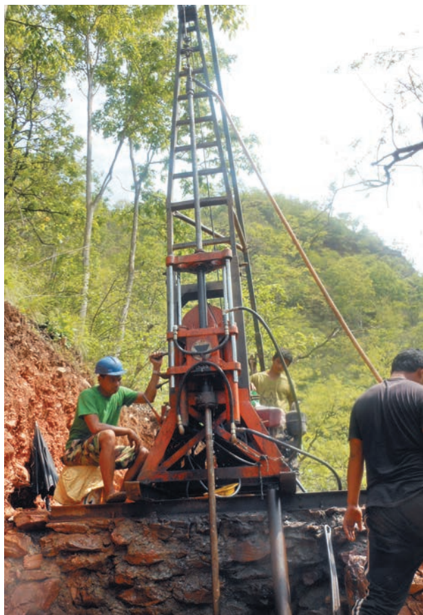
Core Drilling at Dam site
