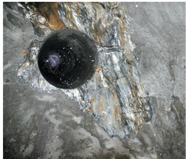
Pilot Shaft for Surge Tank
