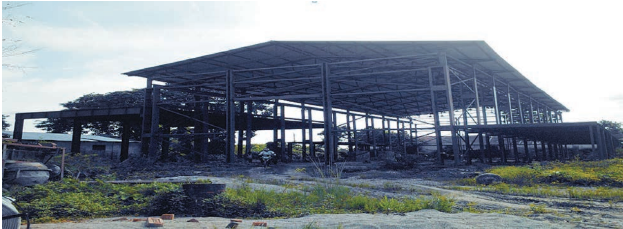
Transformer Testing Lab under construction at Biratnagar Site
