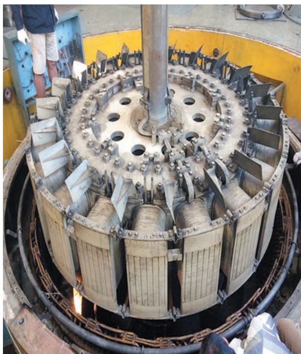
Dismantling of Rotor for Overhauling (Unit #1)
