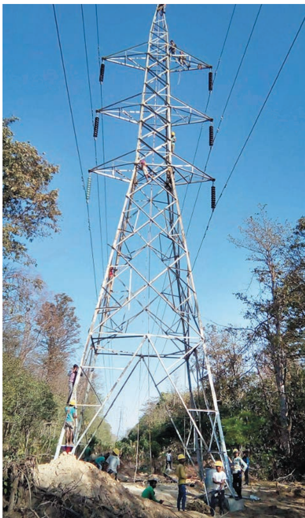
Erection of 132 kV Tower damaged by wild elephants in Kohalpur - Kusum Section
