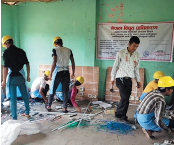
House Wiring Training at Chitwan
