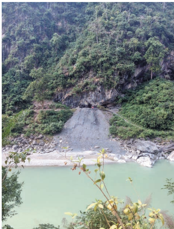
Headworks site of Tanahu HEP
