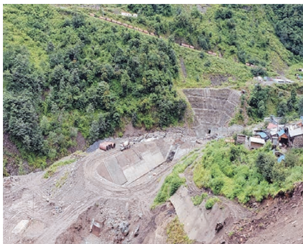
SHEP Headworks- Balancing Pond and Inlet Slope
