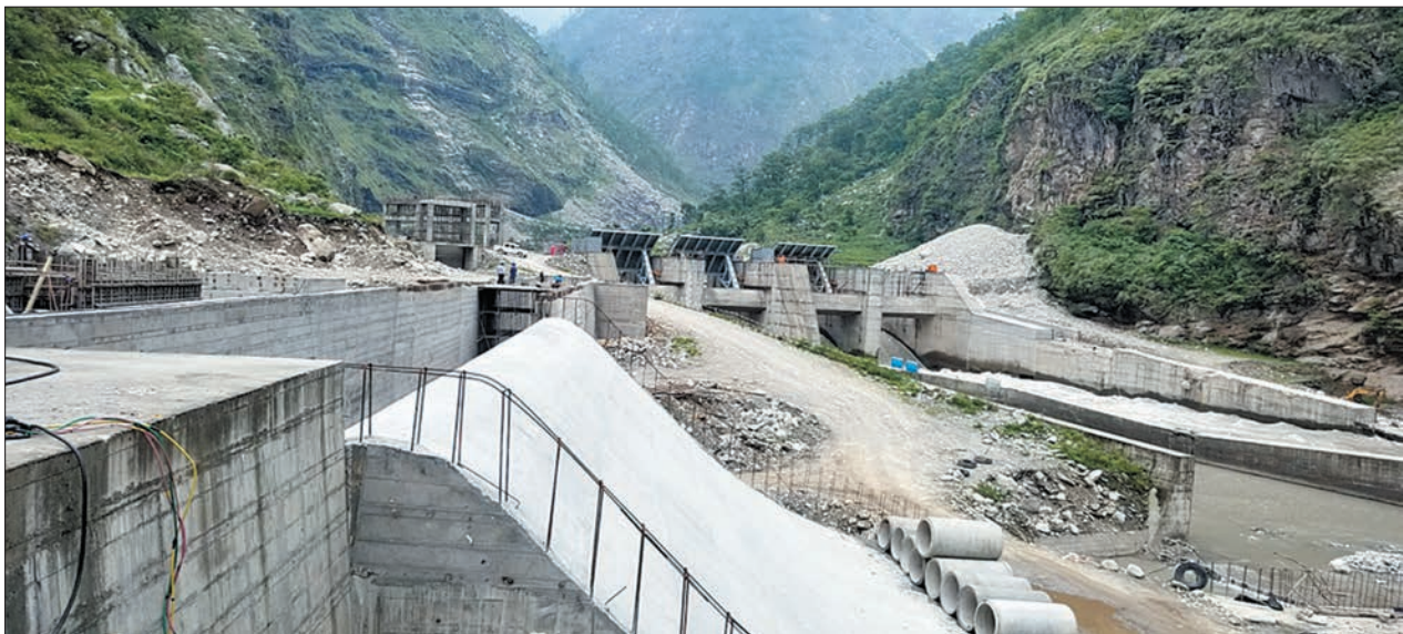
Upper Trishuli 3A Dam Site Area
