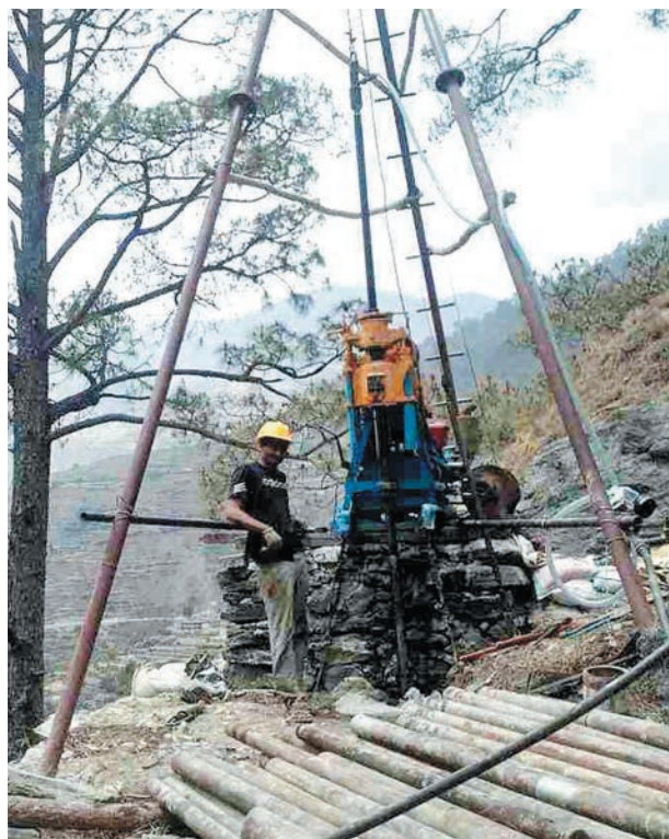
Core drilling works at Upper Modi A, HEP, KASKI
