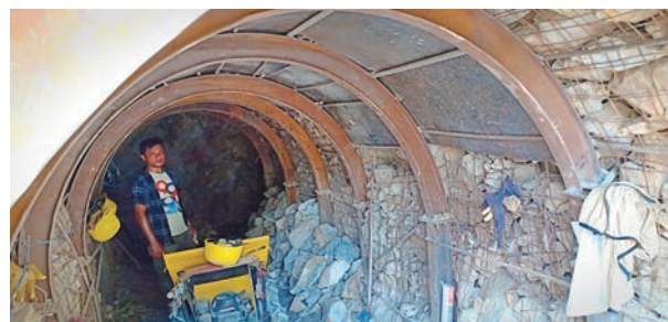
Construction of test adit: Adit no.- AR2
