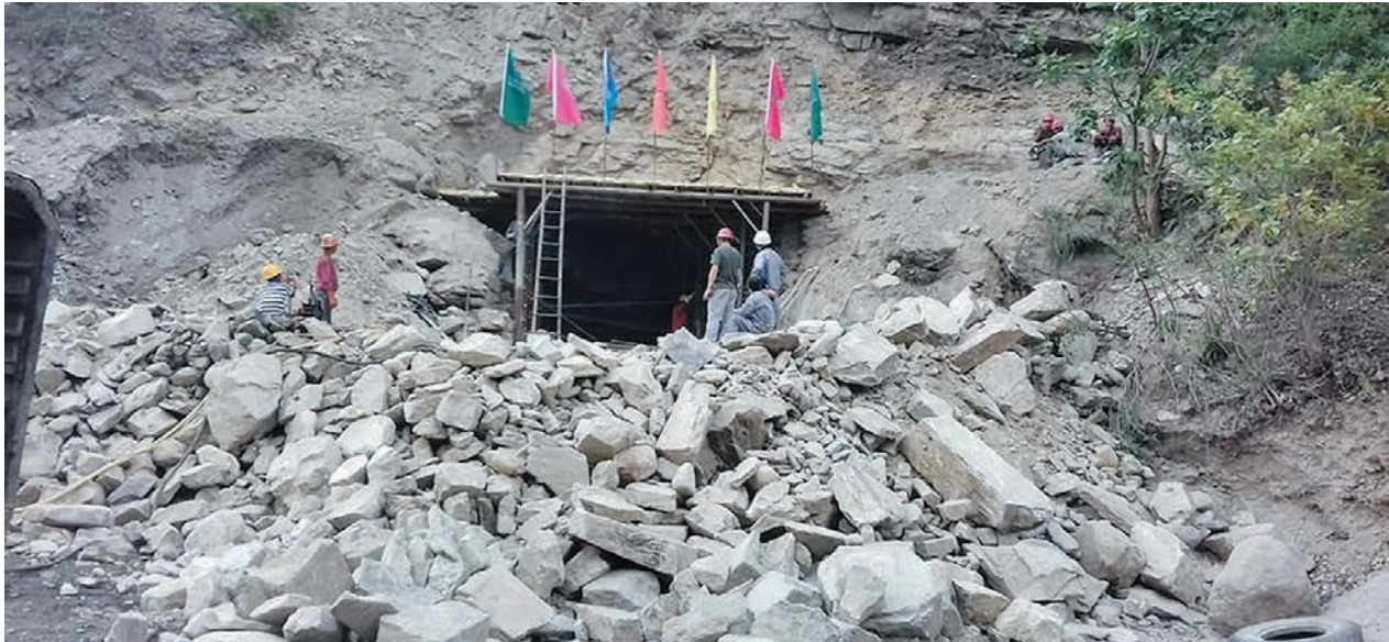
Test Adit Construction
