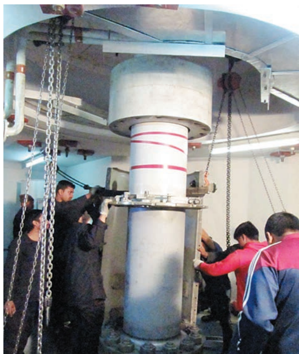
Dismantling of Runner during Overhauling
