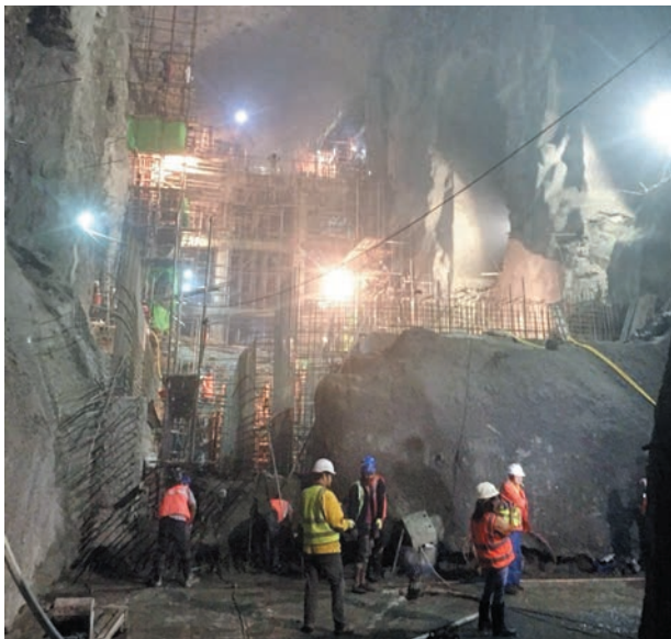
Ongoing works at the powerhouse site.
