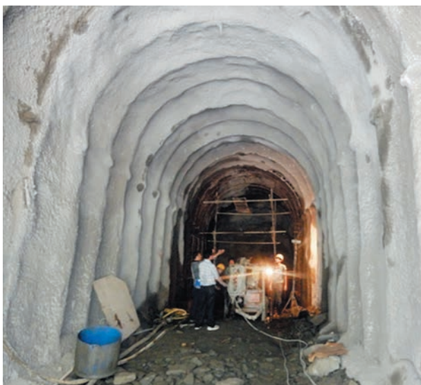
Adit Tunnel to Interconnection
