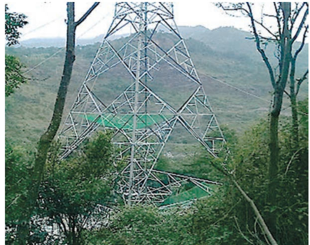
Center line view of 220 kV transmission tower
