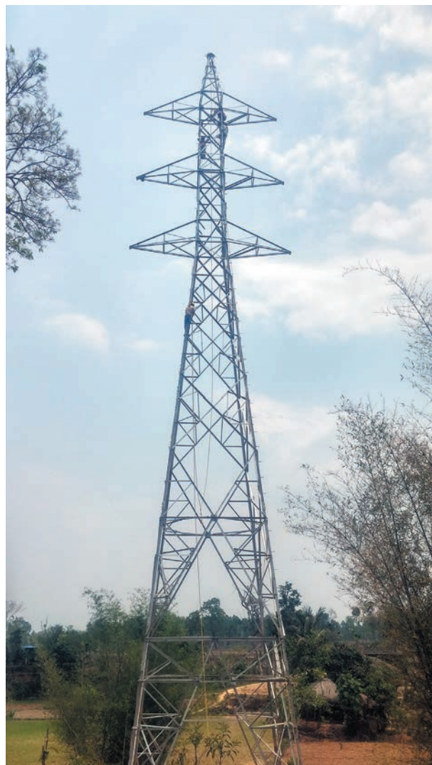
Erection of Tower
