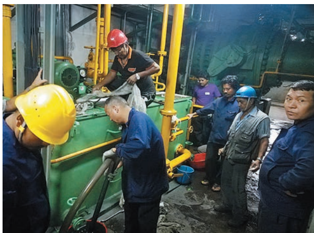
Replacement of Turbine Governor Oil from the Sump
