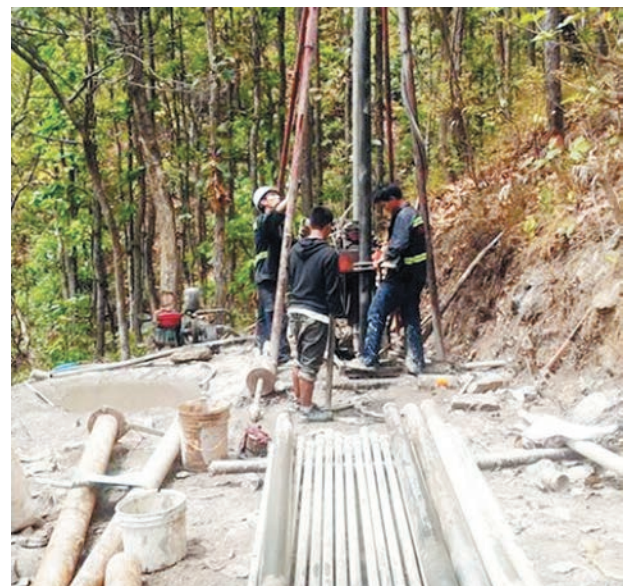
Core Drilling at Surge Tank Area
