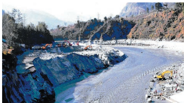
Left Bank Protection Works and Clearance of Sediment from Reservoir and Dam Site
