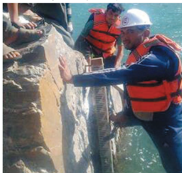
Installation of Gauging Station
