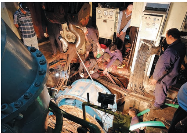
Installation of MIV (Unit #2)
