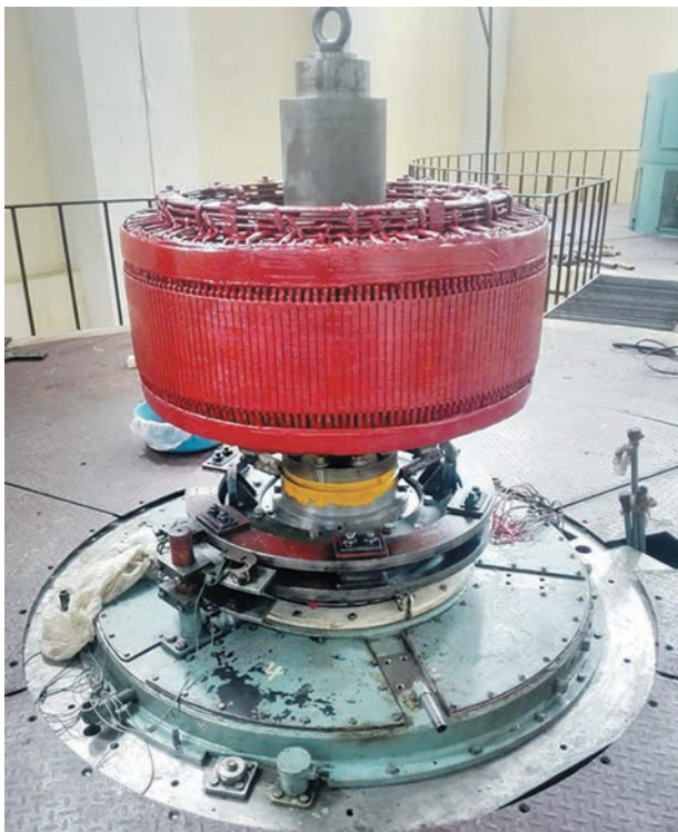
Exciter Rotor (Unit #2)
