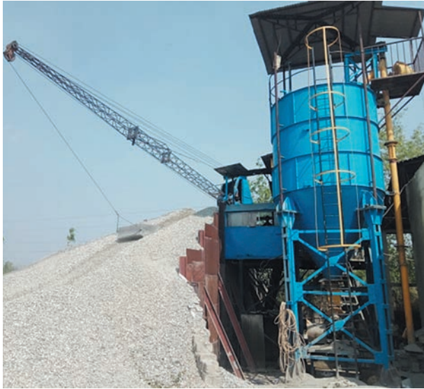
Pole Production at Concrete Pole Plant, Amlekhgunj
