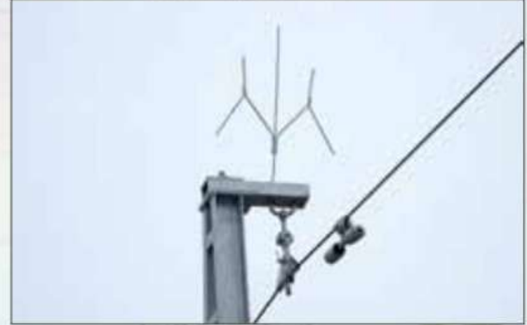
Wishbone Prevents Birds Landing on Wire
