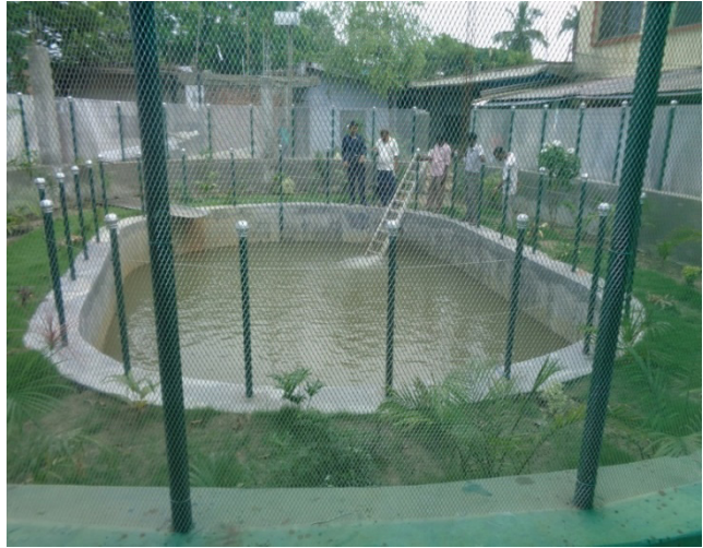
EFLGP supported recharge pond
