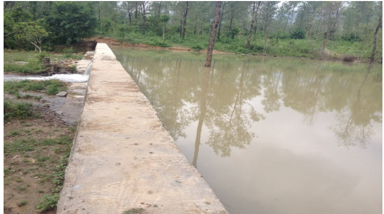
Constructed biological pond
