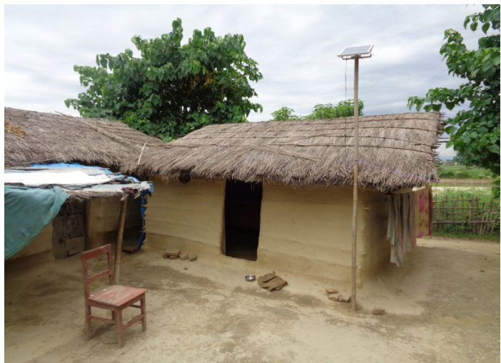
Solar tuki in Kanakpur VDC
