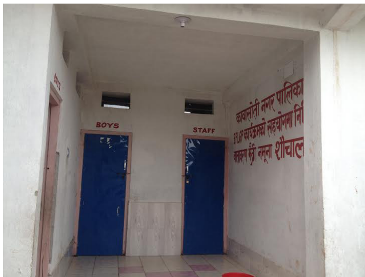
School toilet constructed with attached biogas
