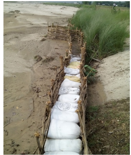
Sand sacks for protection in Jogidaha
