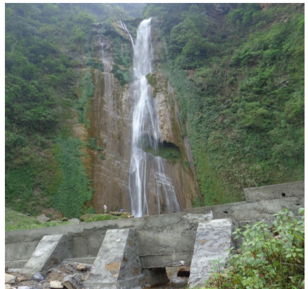
Dam construction from EFLGP
