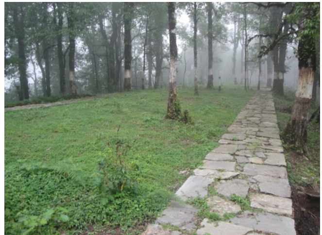
Pavement of footway
