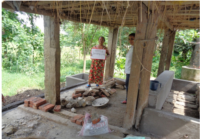
Construction work in progress
