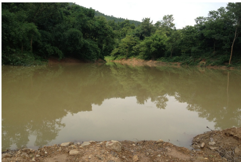
Pond Construction work in Kankai
