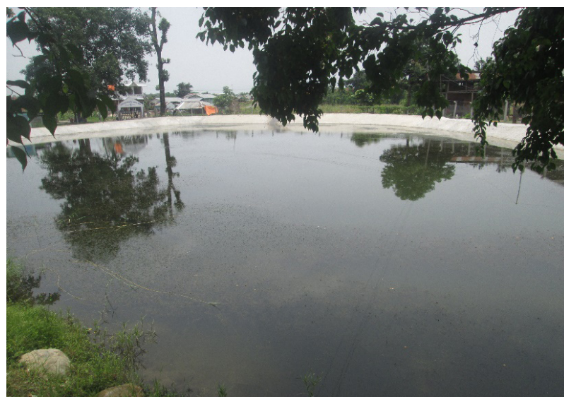
Dhara Pokhari during maintenance
