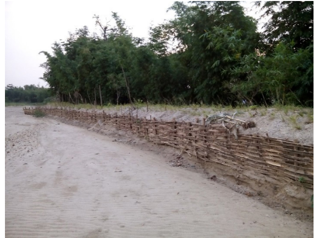
Bamboo retaining wall and plantation work in Jogidaha
