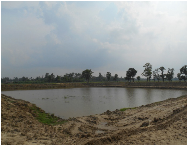
New constructed Dhanusadham Pond
