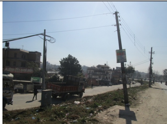
Figure 50. Electric pole no. 38
