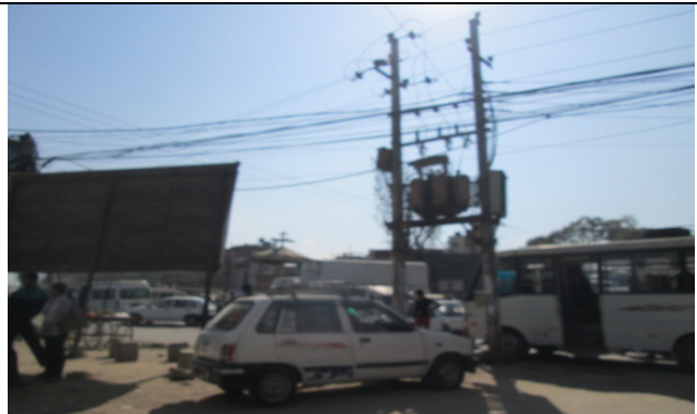
Figure 72. Electric pole no. 52
