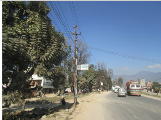
Figure 90. Electric pole no. 88
