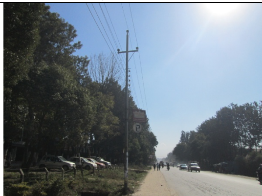
Figure 32. Electric pole no. 19
