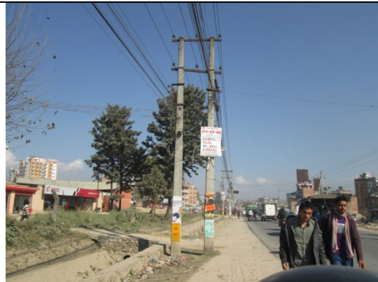
Figure 29. Electric pole no. 14
