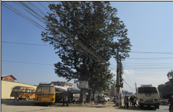
Figure 61. Electric pole no. 38
