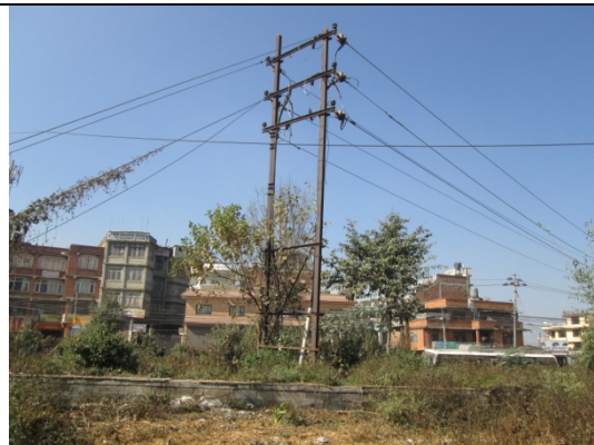
Figure 47. Electric pole no. 40
