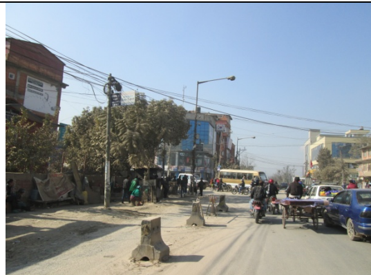
Figure 124. Electric pole no. 122
