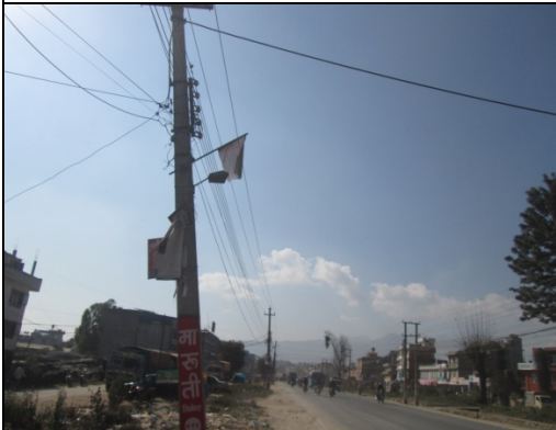
Figure 52. Electric pole no. 37
