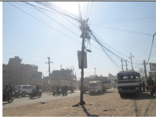
Figure 43. Electric pole no. 36
