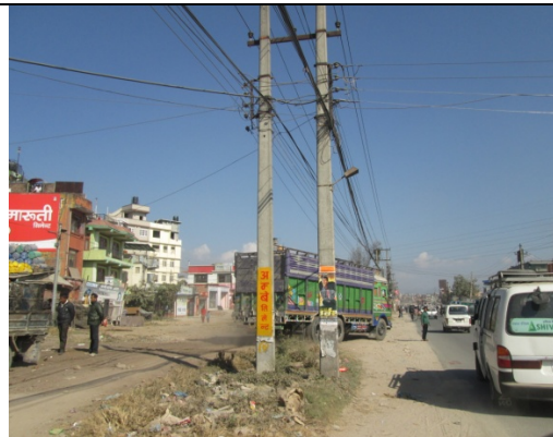
Figure 23. Electric pole no. 8
