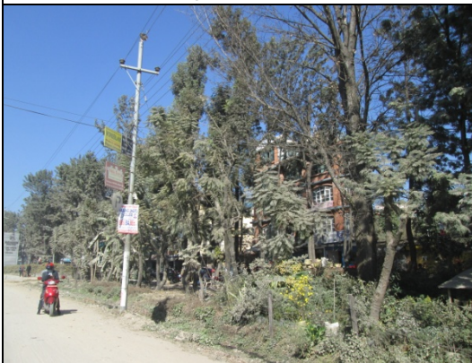
Figure 25. Electric pole no. 12
