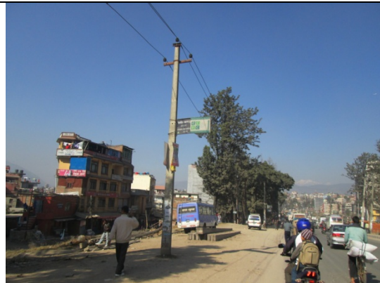
Figure 80. Electric pole no. 77
