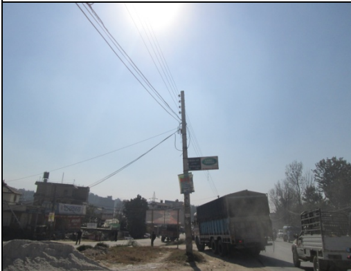
Figure 49. Electric pole no. 37
