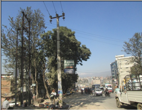
Figure 81. Electric pole no. 78 & 79
