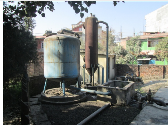
Figure 17. KUKL Water boring plant
