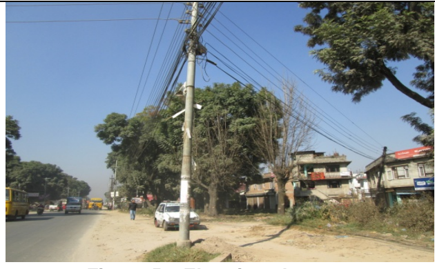
Figure 50. Electric pole no. 26
