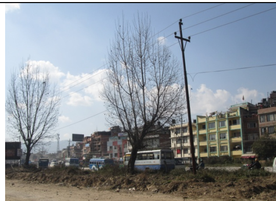
Figure 51. Electric pole no. 44
