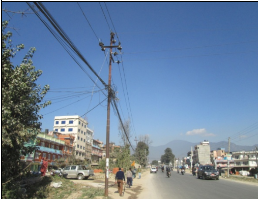
Figure 93. Electric pole no. 91
