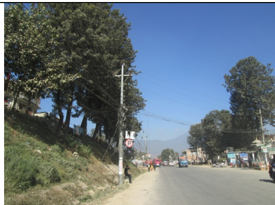
Figure 98. Electric pole no. 96
