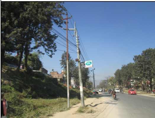
Figure 103. Electric pole no. 101
