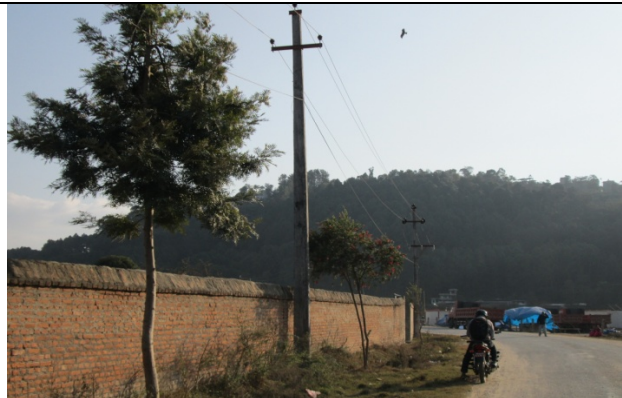
Figure 11. Electric pole no. 16
