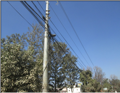
Figure 89. Electric pole no. 87
