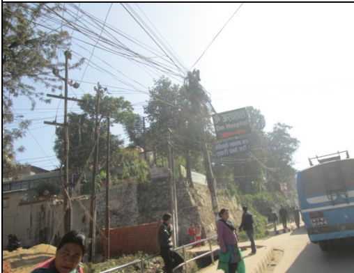
Figure 67. Electric pole no. 61, 62 & 63
