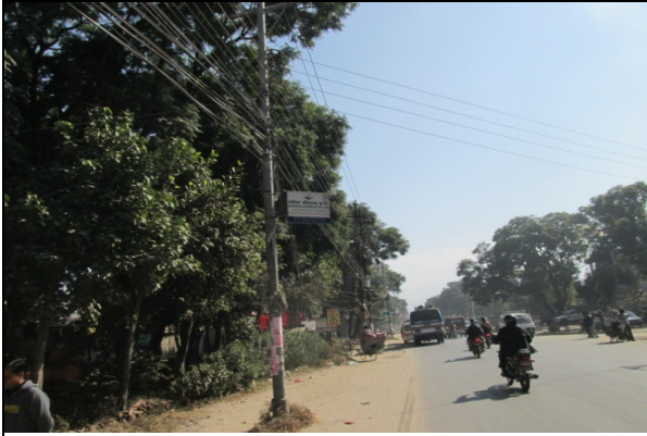
Figure 13. Electric pole no. 21
