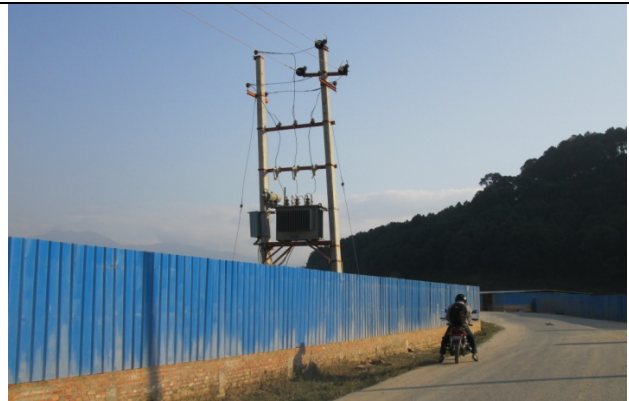
Figure 40. Electric pole no. 22
