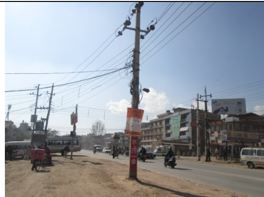
Figure 67. Electric pole no. 53
