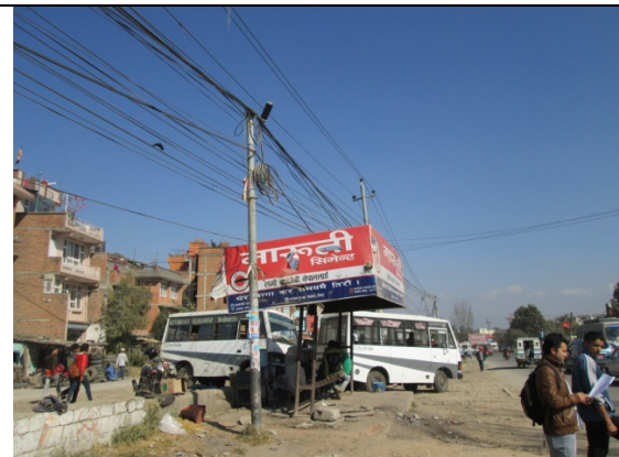
Figure 17. Electric pole no. 3
