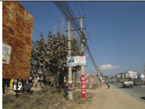
Figure 39. Electric pole no. 24
