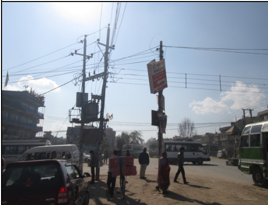
Figure 68. Electric pole no. 54 & 55
