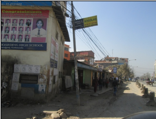
Figure 123. Electric pole no. 121
