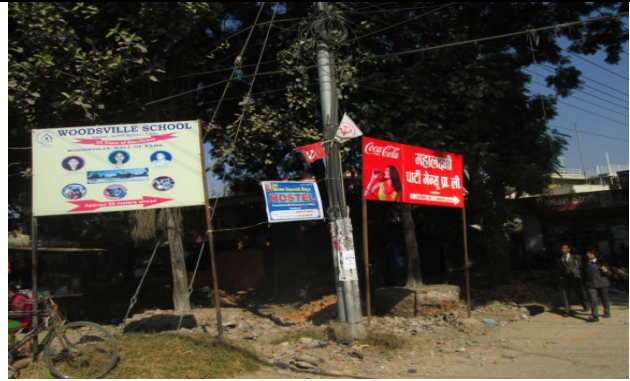
Figure 16. Electric pole no. 24
