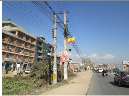
Figure 39. Electric pole no. 29
