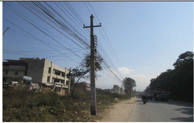
Figure 58. Electric pole no. 35
