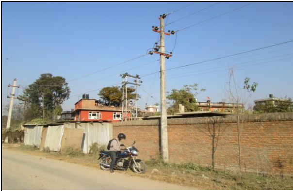
Figure 31. Electric pole no. 13
