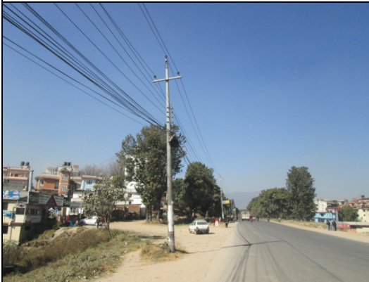
Figure 111. Electric pole no. 109
