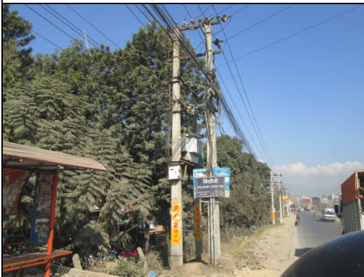
Figure 34. Electric pole no. 24
