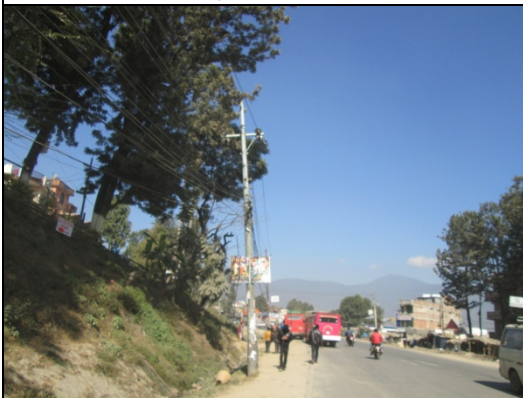
Figure 99. Electric pole no. 97
