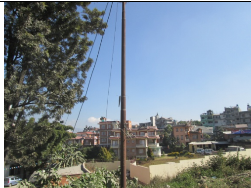
Figure 38. Electric pole no. 25
