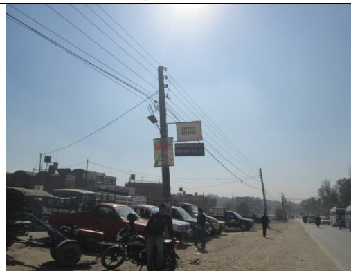
Figure 46. Electric pole no. 34
