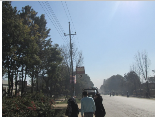
Figure 30. Electric pole no. 17
