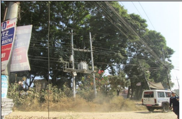
Figure 41. Electric pole no. 17
