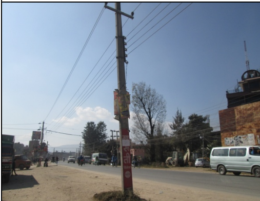
Figure 44. Electric pole no. 29
