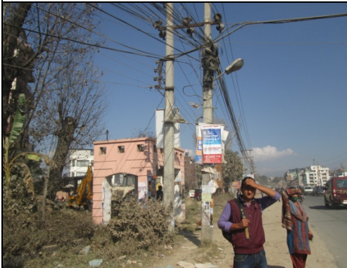
Figure 38. Electric pole no. 23
