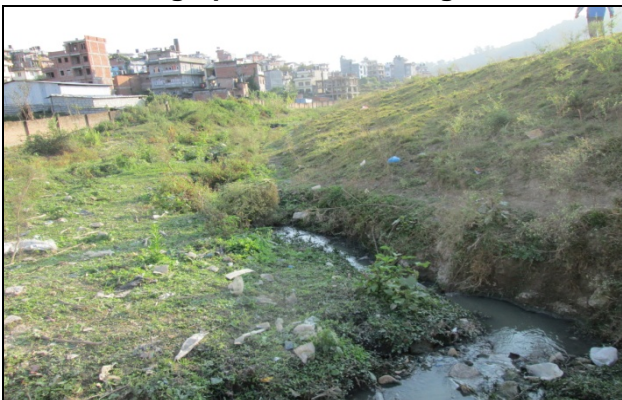
Figure 41. Surface sewer and storm water drain inlet
