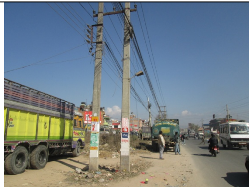
Figure 21. Electric pole no. 6
