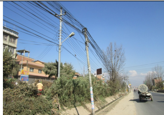
Figure 25. Electric pole no. 11 & 12
