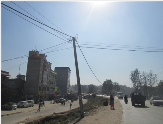
Figure 55. Electric pole no. 44
