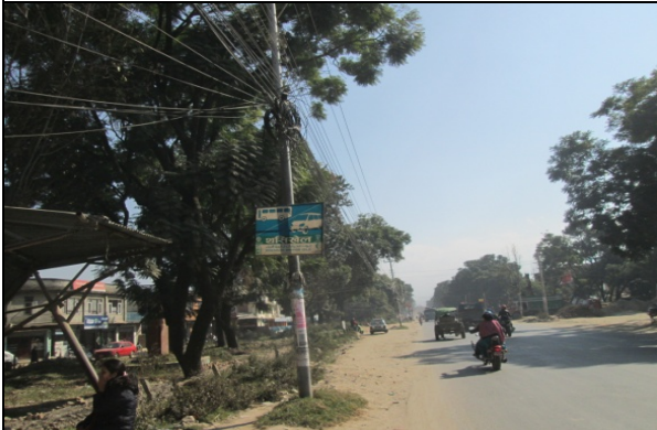
Figure 17. Electric poles no. 25
