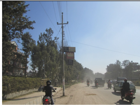
Figure 24. Electric pole no. 11
