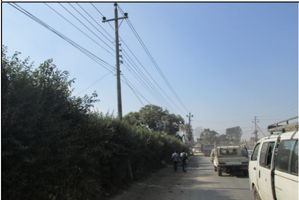
Figure 46. Electric pole no. 92
