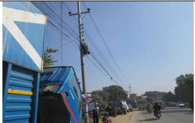
Figure 9. Electric pole no. 12
