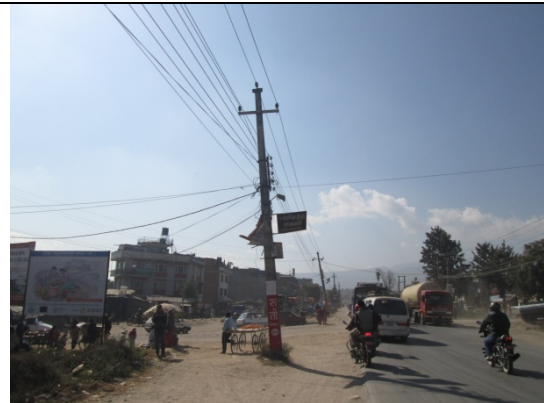
Figure 51. Electric pole no. 36
