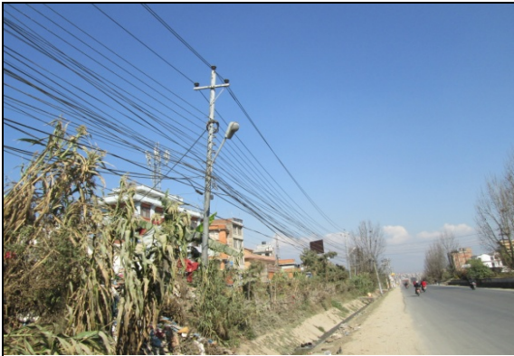
Figure 24. Electric pole no. 10
