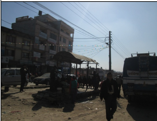
Figure 45. Electric pole no. 33
