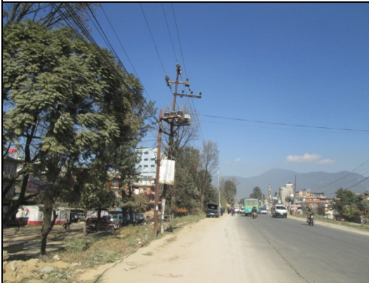
Figure 91. Electric pole no. 89
