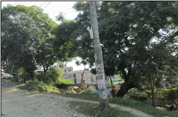
Figure 97. Electric pole no. 78
