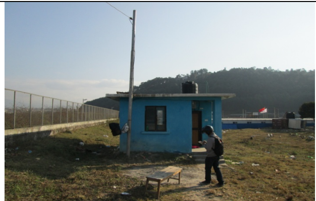
Figure 7. Electric pole no. 10
