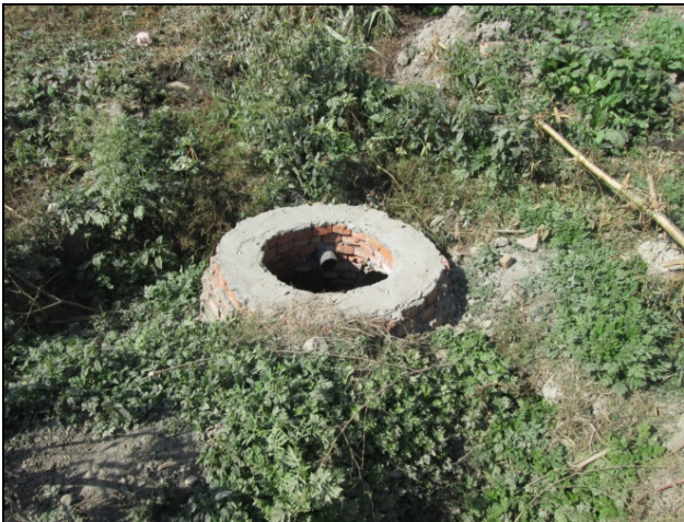
Figure 15. Inlet of underground sewer
