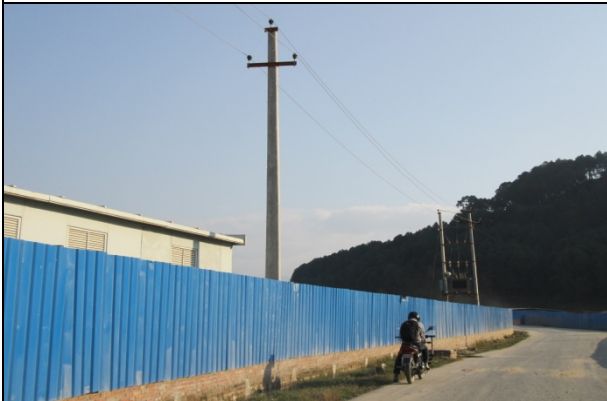
Figure 16. Electric pole no. 21
