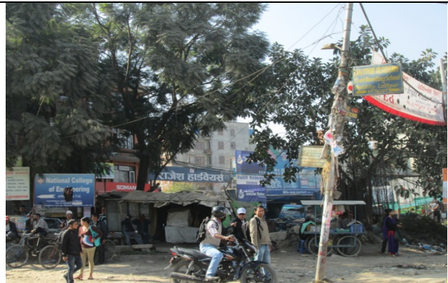
Figure 82. Electric pole no. 62
