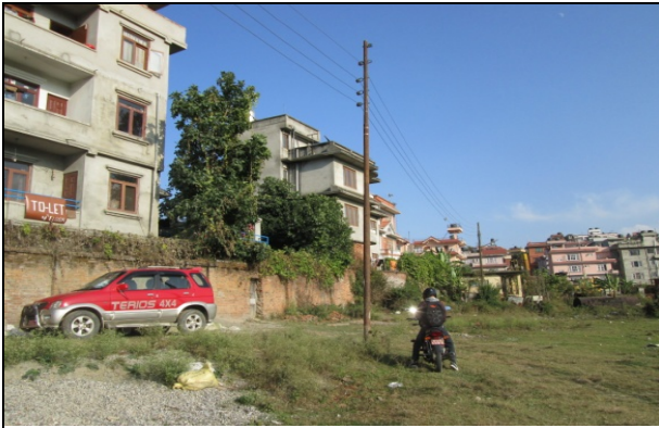
Figure 4. Electric pole no. 7
