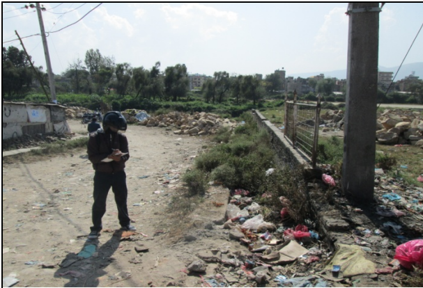
Figure 8. Inlet of Storm water drain no. 4
