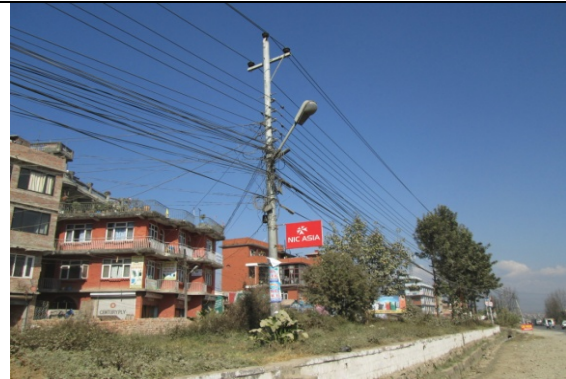
Figure 21. Electric pole no. 7
