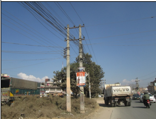
Figure 34. Electric pole no. 19
