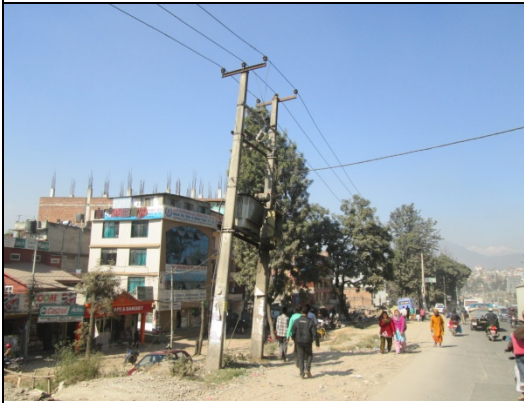
Figure 79. Electric pole no. 76
