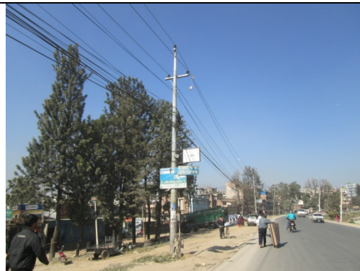
Figure 86. Electric pole no. 84
