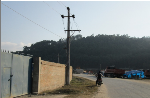
Figure 12. Electric pole no. 17
