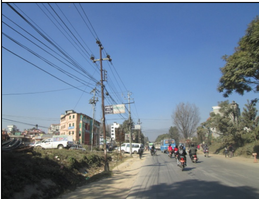
Figure 109. Electric pole no. 107
