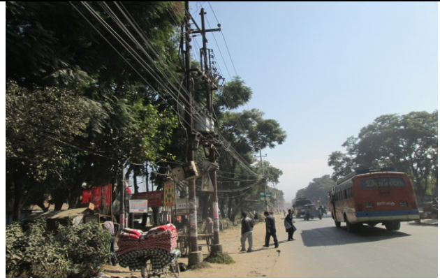
Figure 14. Electric pole no. 22
