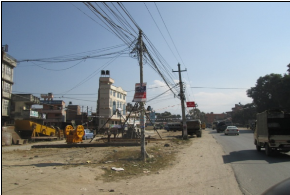
Figure 63. Electric pole no. 40 & 41
