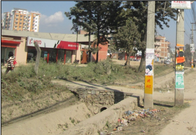
Figure 69. Surface storm water drain along road
