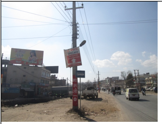
Figure 64. Electric pole no. 50
