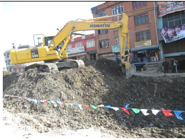
Figure 72. Construction activities in front of Gopi Krishna Hall
