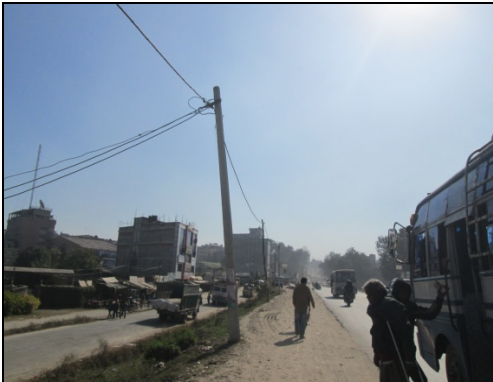
Figure 59. Electric pole no. 48
