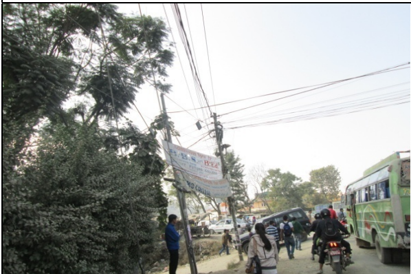
Figure 48. Electric pole no. 94
