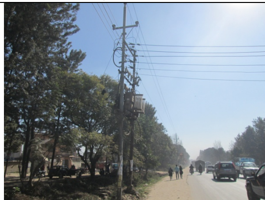
Figure 28. Electric pole no. 15
