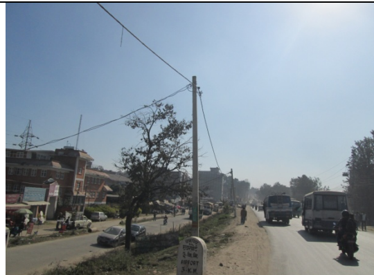
Figure 58. Electric pole no. 47
