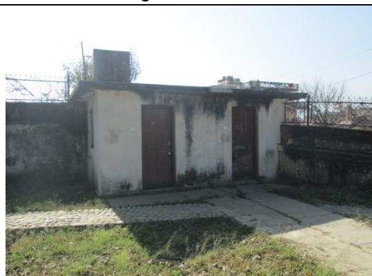
Figure 13. Temporary Bus stand
