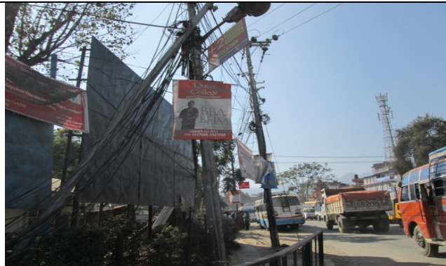
Figure 24. Electric pole no. 54
