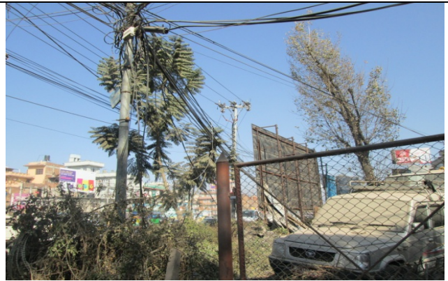
Figure 26. Electric pole no. 56
