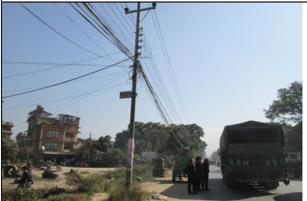
Figure 43. Electric pole no. 19
