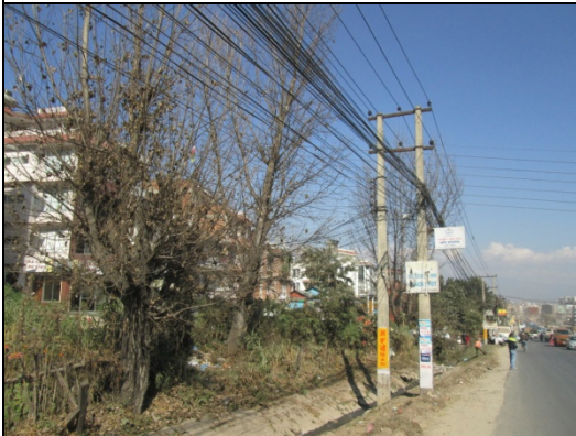
Figure 32. Electric pole no. 22
