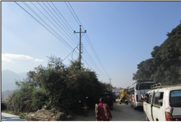
Figure 44. Electric pole no. 90
