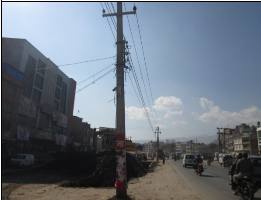
Figure 62. Electric pole no. 48
