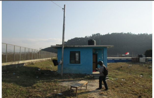
Figure 50. Building of solar Energy (no. 6)
