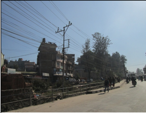
Figure 65. Electric pole no. 59
