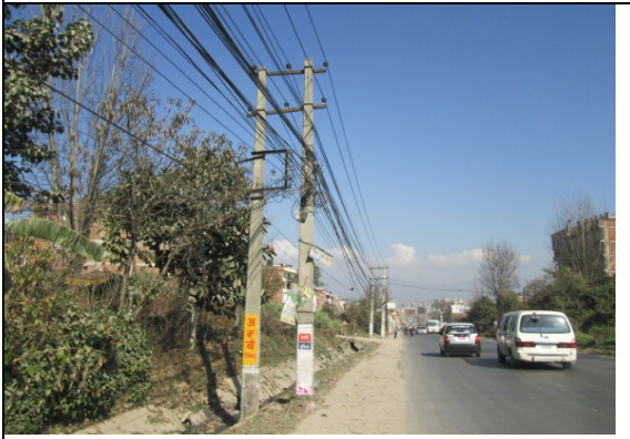
Figure 28. Electric pole no. 18
