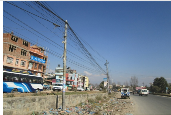
Figure 19. Electric pole no. 5
