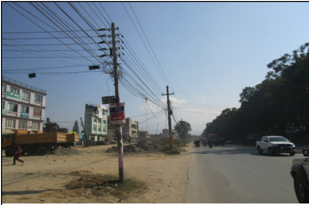
Figure 57. Electric pole no. 33 & 34
