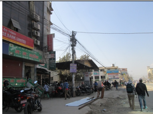
Figure 122. Electric pole no. 120
