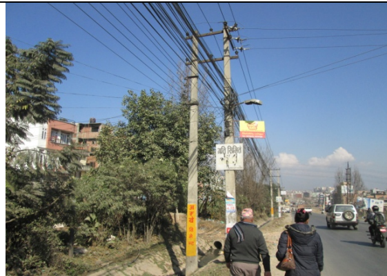
Figure 31. Electric pole no. 21
