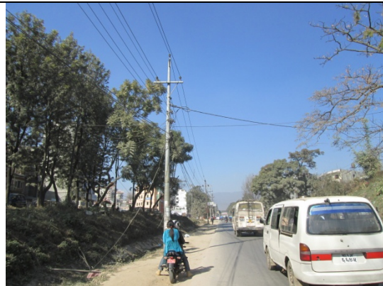
Figure 108. Electric pole no. 106
