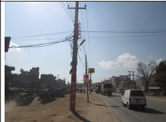
Figure 65. Electric pole no. 51
