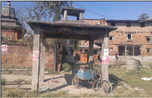
Figure 10. Unused Cremation area no 1
