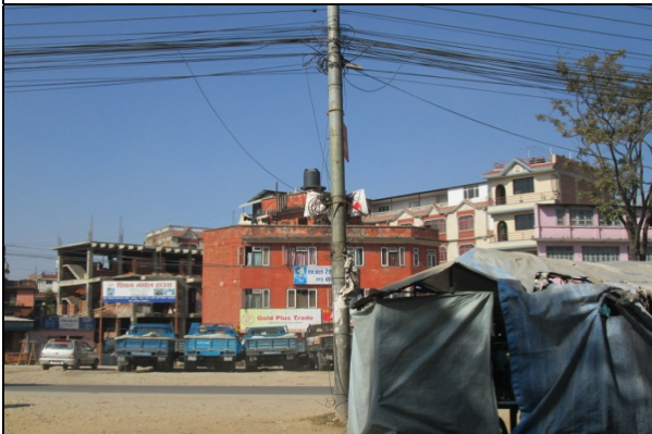
Figure 29. Electric pole no. 59
