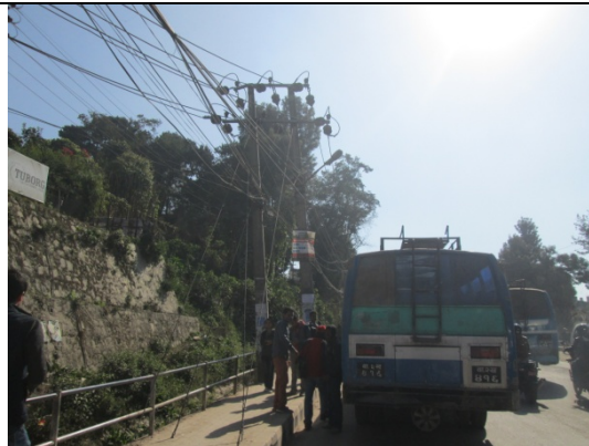
Figure 68. Electric pole no. 64
