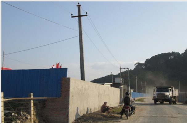
Figure 14. Electric pole no. 19
