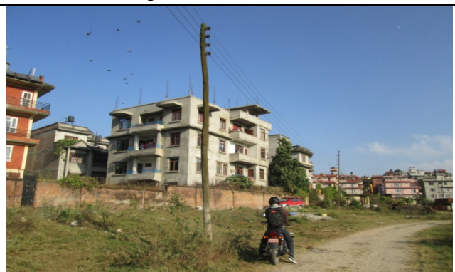
Figure 3. Electric pole no. 6
