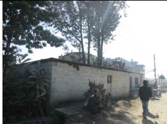
Figure 151. Traffic police post
