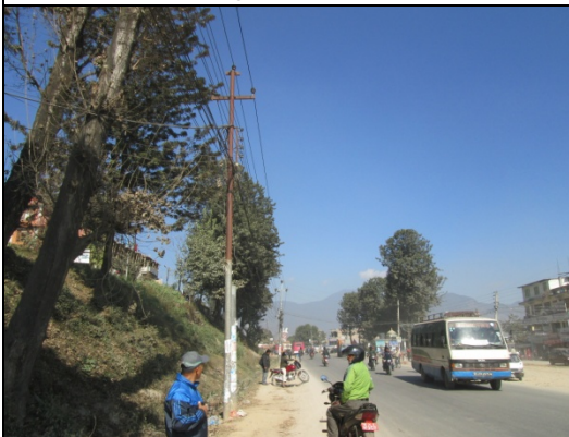
Figure 97. Electric pole no. 95
