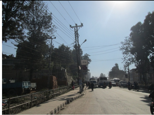
Figure 66. Electric pole no. 60
