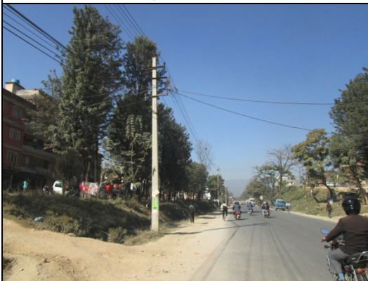
Figure 105. Electric pole no. 103
