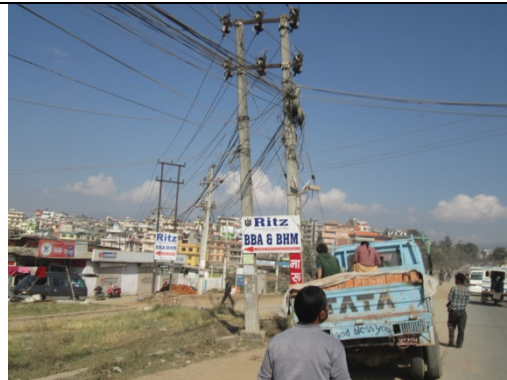
Figure 41. Electric pole no. 26
