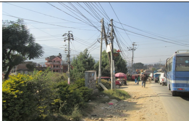
Figure 100. Electric pole no. 81 , 82 & 83
