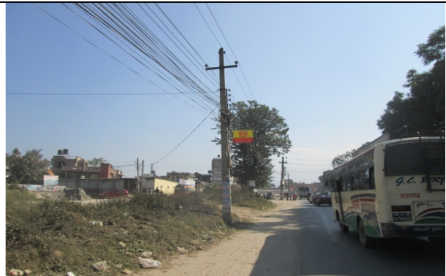
Figure 60. Electric pole no. 37
