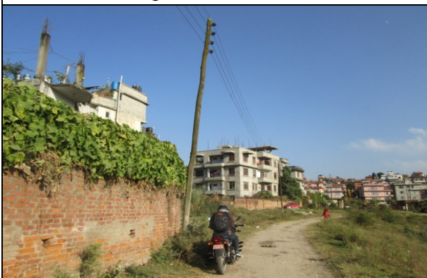
Figure 2. Electric pole no. 5
