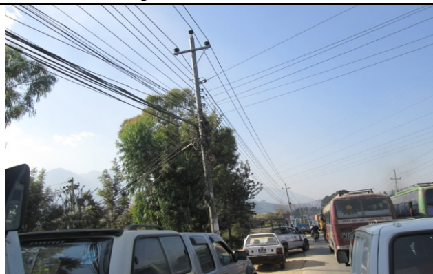
Figure 102. Electric pole no. 85
