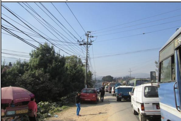
Figure 101. Electric pole no. 84
