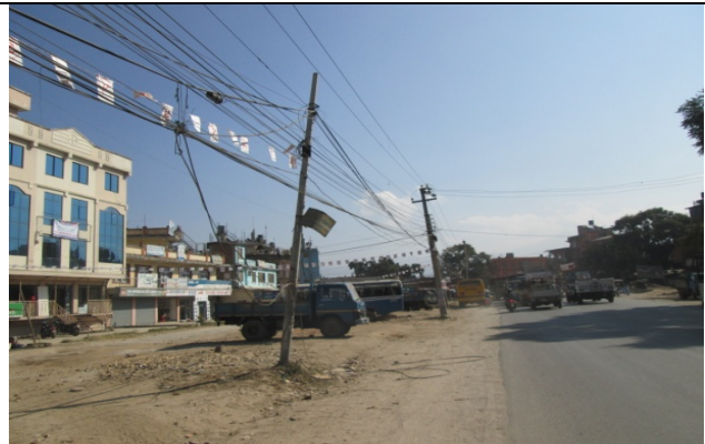
Figure 18. Electric pole no. 42 & 43
