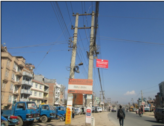
Figure 16. Electric pole no. 1
