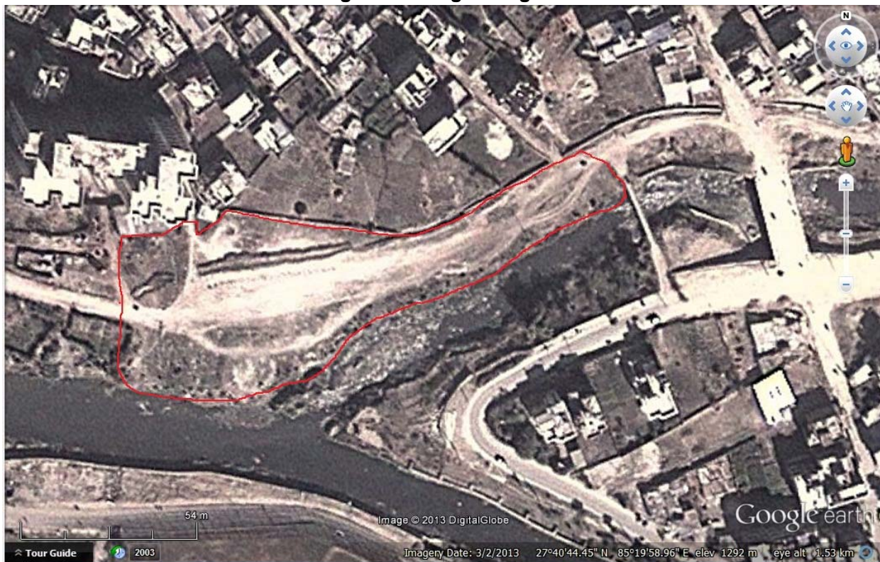
Figure 1. Google Image of site
