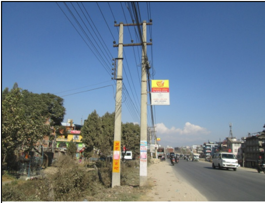
Figure 36. Electric pole no. 26
