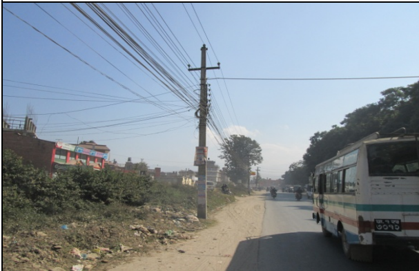
Figure 59. Electric pole no. 36
