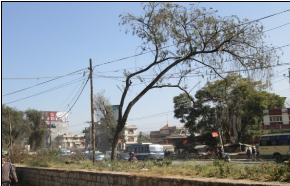
Figure 23. Electric pole no. 48
