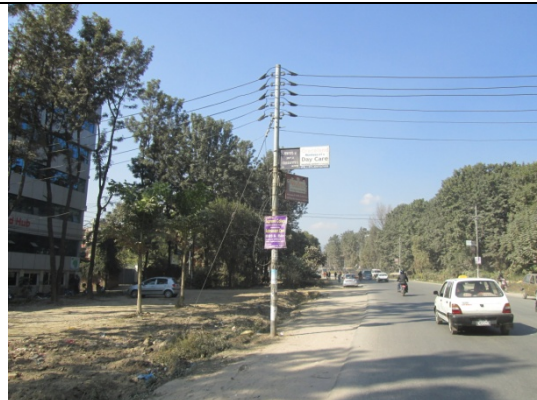
Figure 120. Electric pole no. 118
