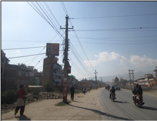
Figure 48. Electric pole no. 33
