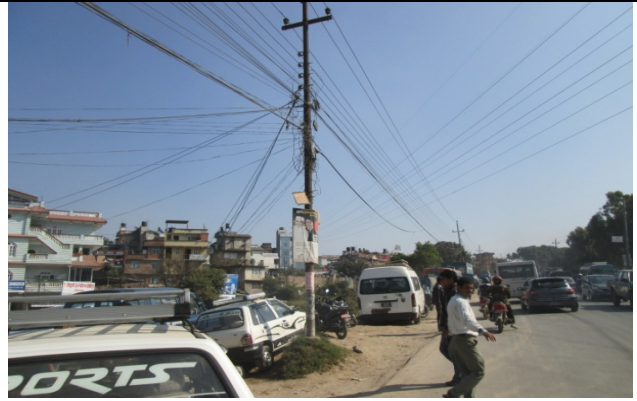
Figure 7. Electric pole no. 11
