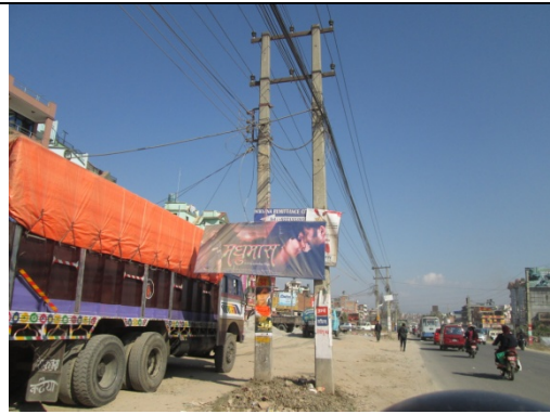
Figure 19. Electric pole no. 4
