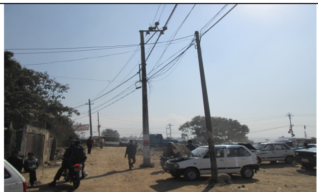
Figure 3. Electric pole no. 2 & 3
