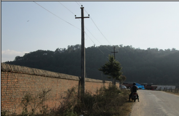
Figure 10. Electric pole no. 15
