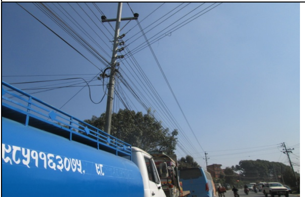
Figure 10. Electric pole no. 13
