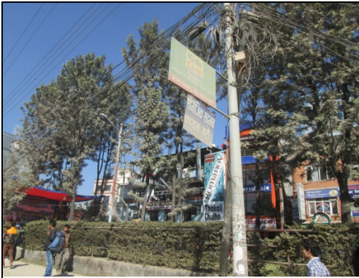
Figure 23. Electric pole no. 10
