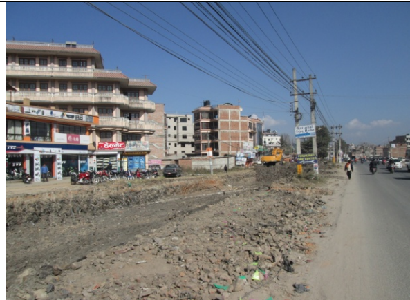
Figure 70. Construction activities along the road
