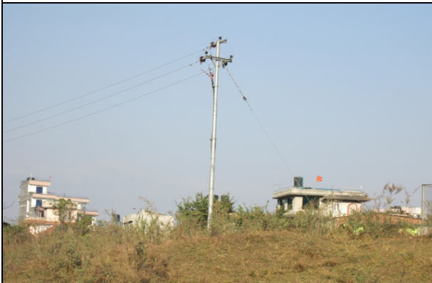
Figure 8. Electric pole no. 11
