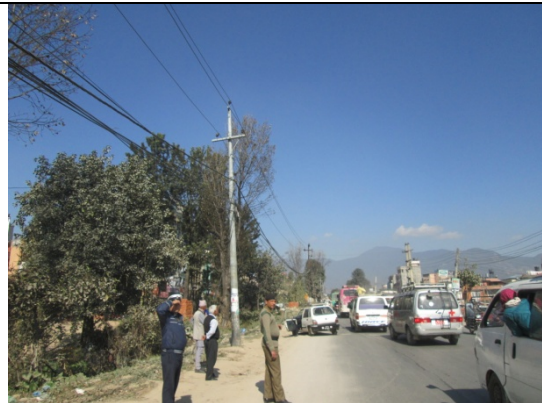
Figure 92. Electric pole no. 90
