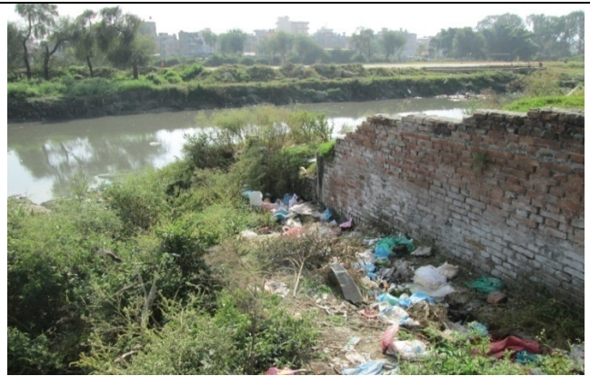
Figure 9. Outlet of Storm water drain no. 4
