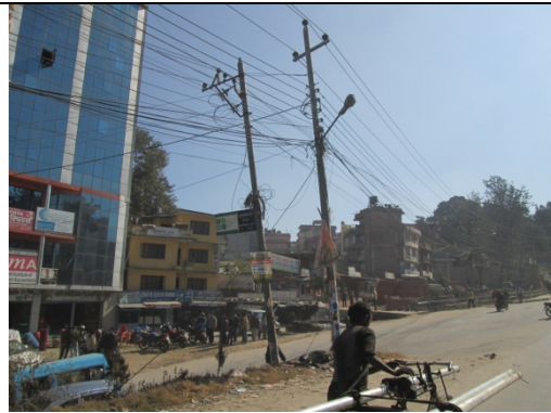
Figure 64. Electric pole no. 57 & 58
