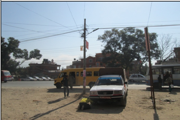
Figure 21. Electric pole no. 46
