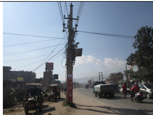
Figure 47. Electric pole no. 32
