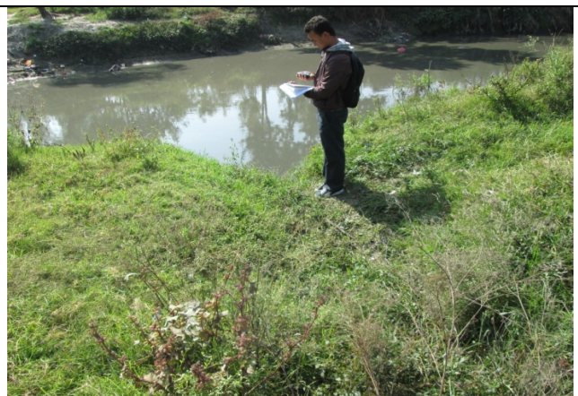
Figure 12. Outlet of Surface Storm water drainage no. 1 and underground sewer no. 1
