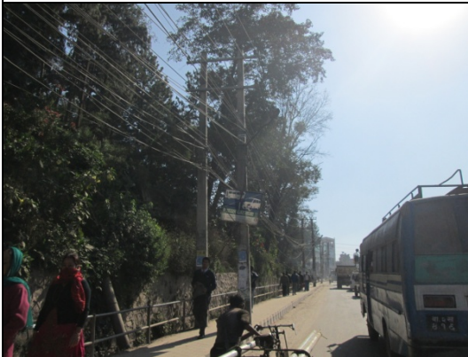
Figure 69. Electric pole no. 65
