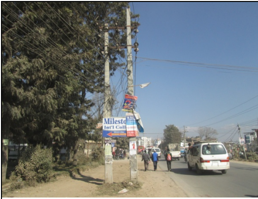
Figure 36. Electric pole no. 21
