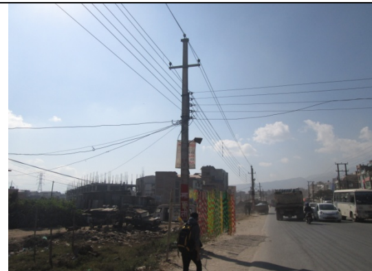
Figure 59. Electric pole no. 45
