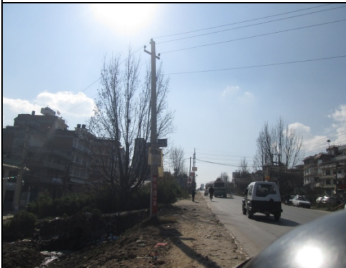
Figure 44. Electric pole no. 37
