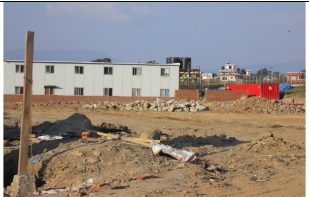
Figure 52. Office Building of Chinese ring road expansion team (no. 8)
