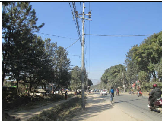
Figure 116. Electric pole no. 114
