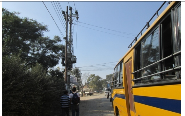
Figure 47. Electric pole no. 93
