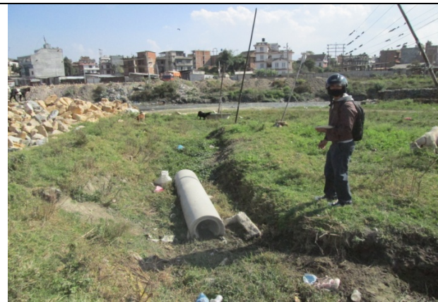
Figure 8. Storm water drain outlet
