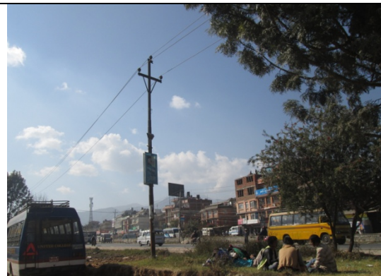
Figure 53. Electric pole no. 46
