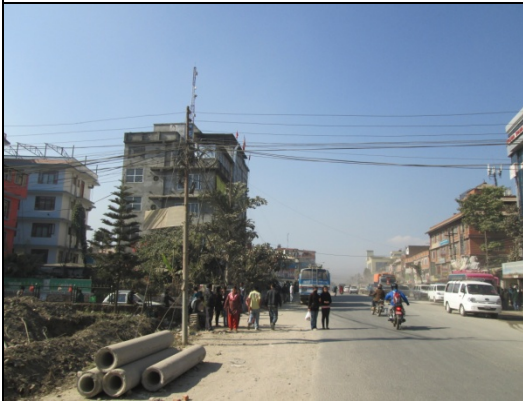
Figure 121. Electric pole no. 119
