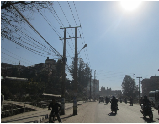
Figure 71. Electric pole no. 67
