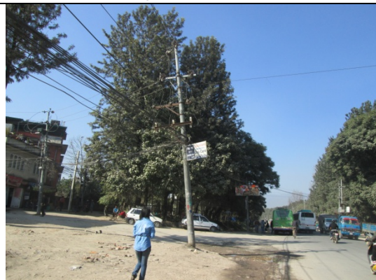
Figure 118. Electric pole no. 116
