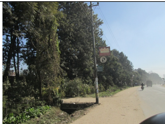
Figure 26. Electric pole no. 13
