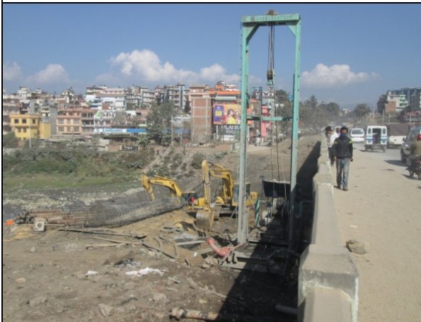
Figure 71. Construction activities along the road in the Balkumari Bridge
