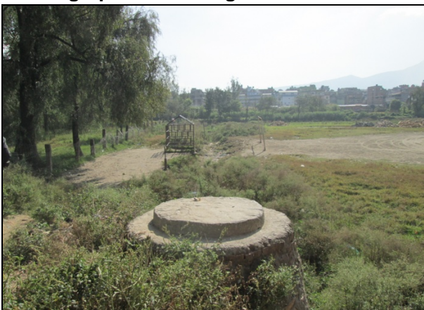
Figure 11. Inlet of Surface Storm water drainage no. 1 and underground sewer no. 1
