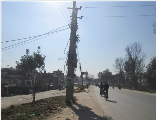
Figure 51. Electric pole no. 39
