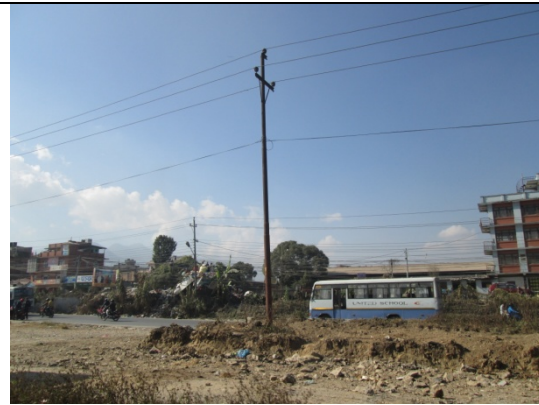
Figure 49. Electric pole no. 42
