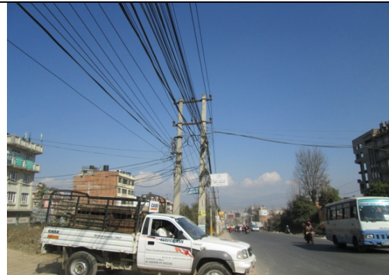
Figure 29. Electric pole no. 19
