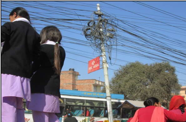
Figure 27. Electric pole no. 57
