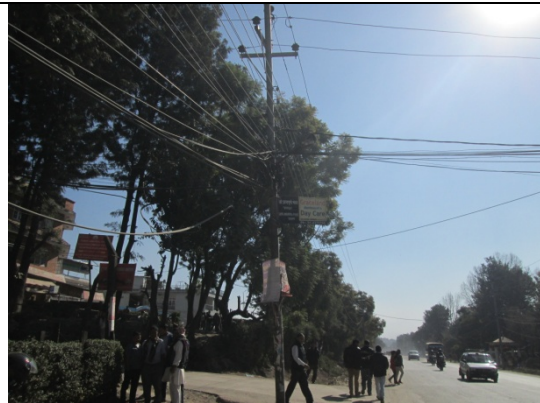
Figure 36. Electric pole no. 23
