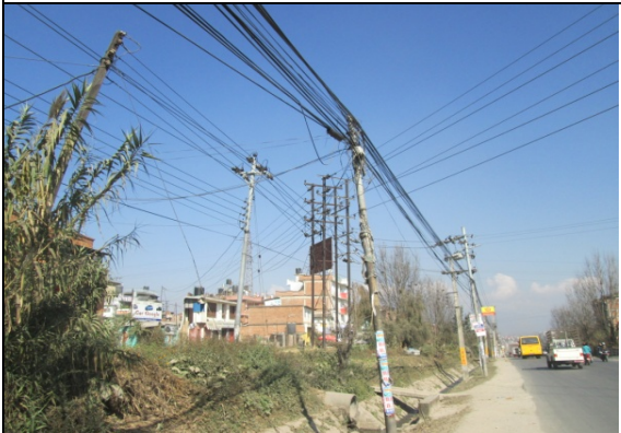
Figure 26. Electric pole no. 13, 14, 15 & 16
