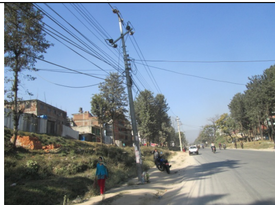
Figure 104. Electric pole no. 102
