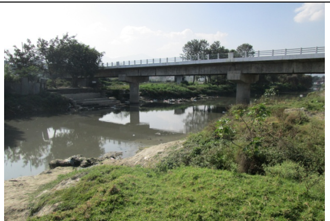
Figure 1. Outlet of Surface Storm water drainage no. 2 and sewer no. 2
