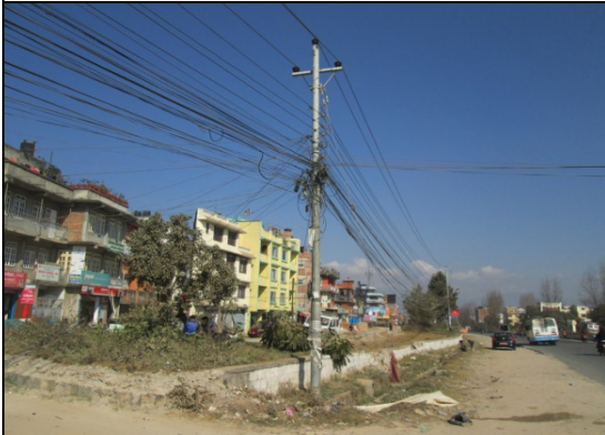
Figure 20. Electric pole no. 6
