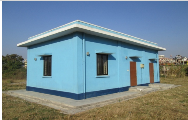
Figure 23. Office Building of solar Energy (no. 4)
