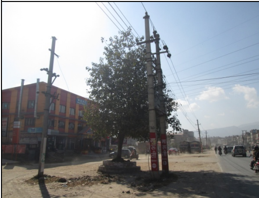
Figure 56. Electric pole no. 41 & 42
