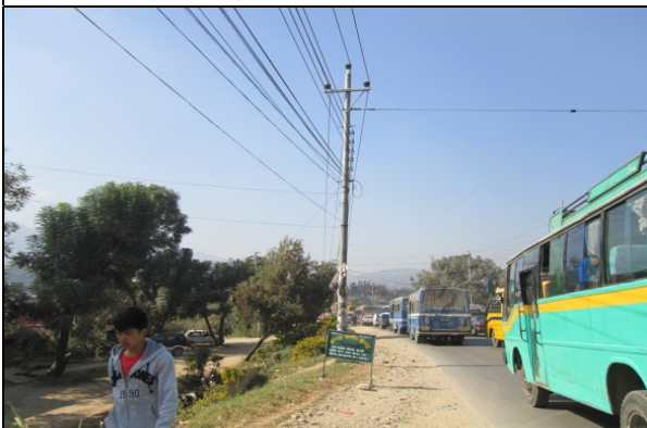
Figure 99. Electric pole no. 80
