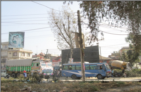
Figure 71. Electric poles no. 51
