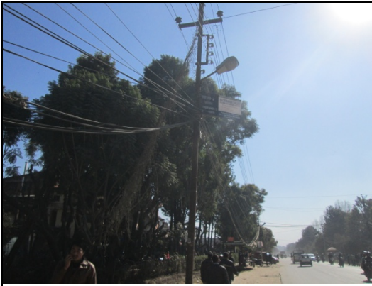
Figure 35. Electric pole no. 22
