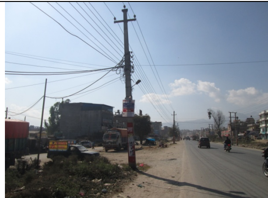
Figure 53. Electric pole no. 38
