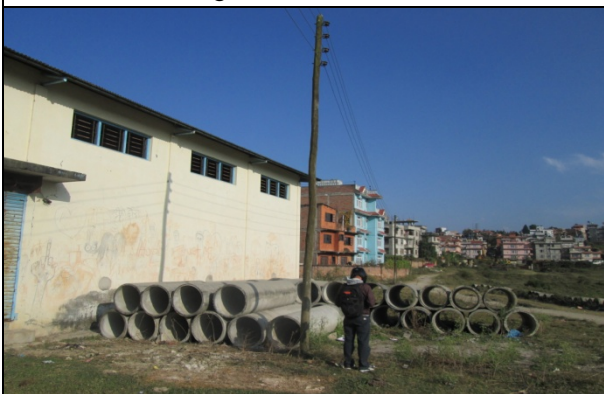
Figure 21. Electric poles no. 3
