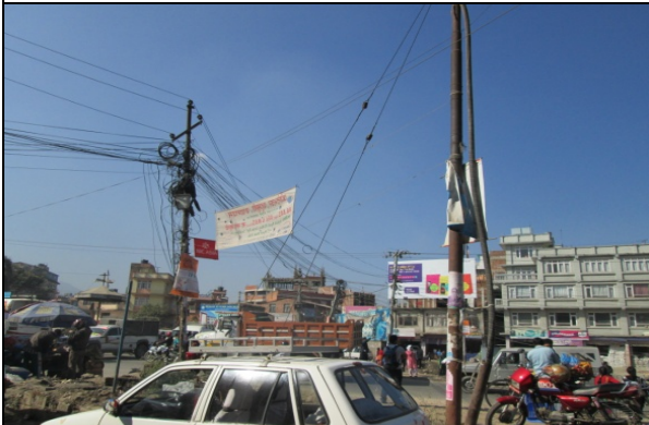
Figure 73. Electric pole no. 53
