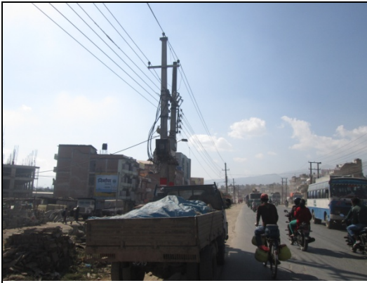
Figure 60. Electric pole no. 46
