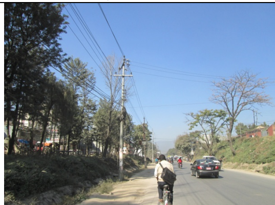
Figure 106. Electric pole no. 104
