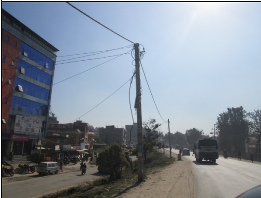
Figure 57. Electric pole no. 46
