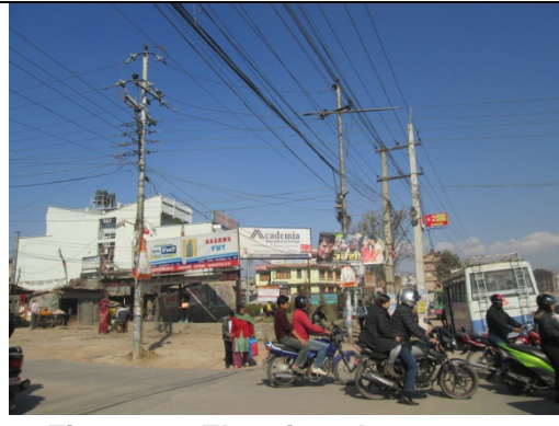
Figure 41. Electric pole no. 31, 32, 33 & 34
