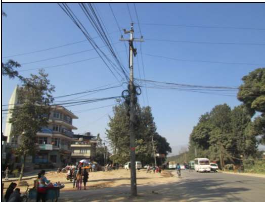
Figure 117. Electric pole no. 115
