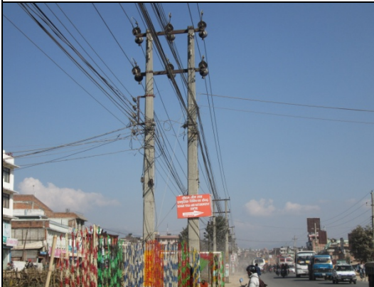
Figure 26. Electric pole no. 11
