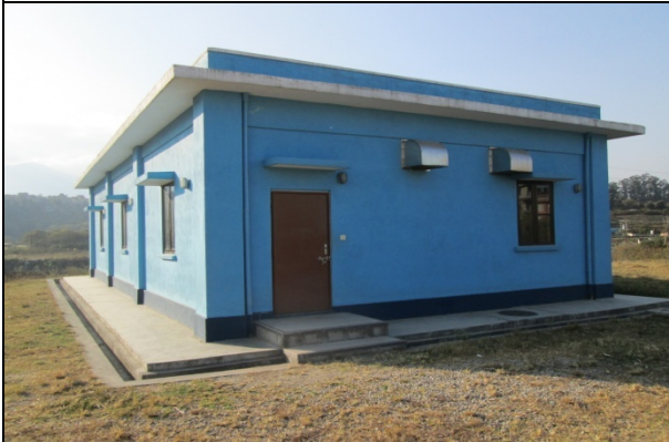
Figure 24. Office Building of solar Energy (no. 5)
