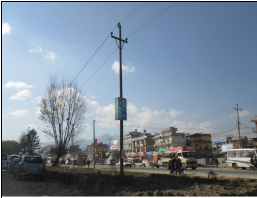
Figure 54. Electric pole no. 47
