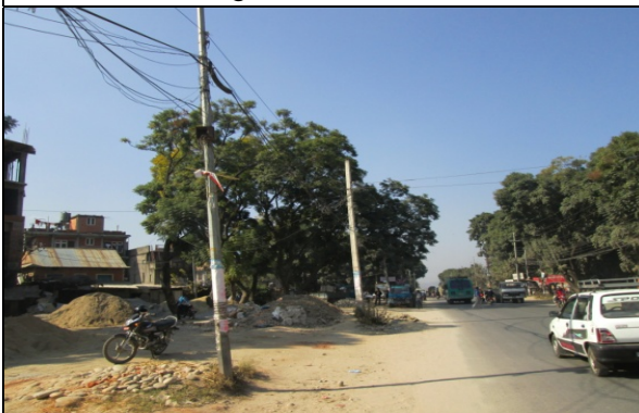
Figure 91. Electric pole no. 71 & 72
