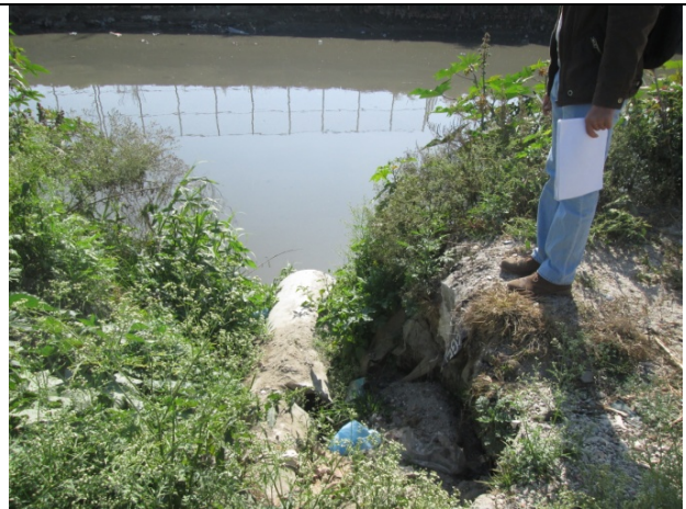
Figure 16. Outlet of underground sewer
