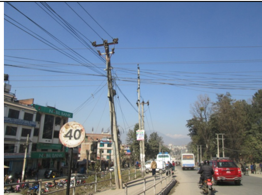
Figure 78. Electric pole no. 74 & 75
