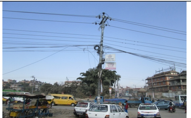
Figure 49. Electric pole no. 95
