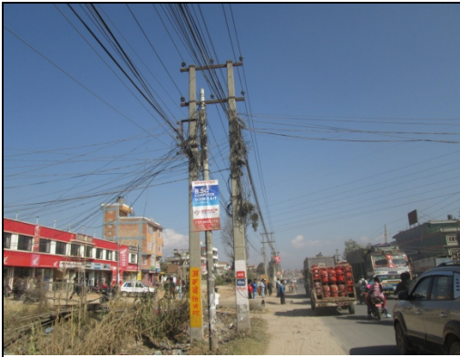
Figure 24. Electric pole no. 9
