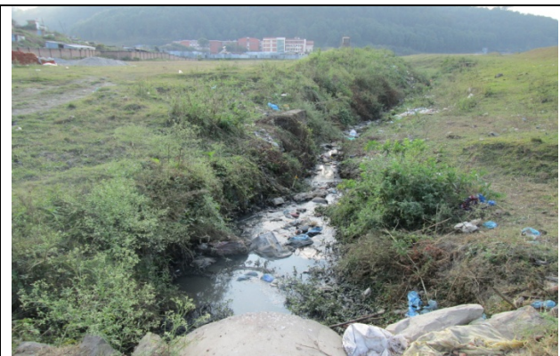
Figure 17. Surface sewer and storm water drain mid point
