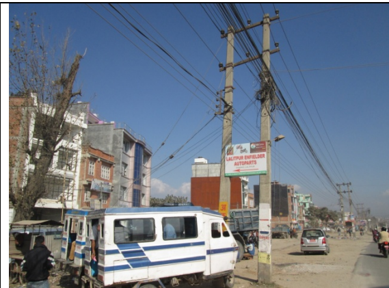
Figure 17. Electric pole no. 2
