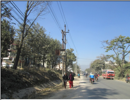
Figure 107. Electric pole no. 105
