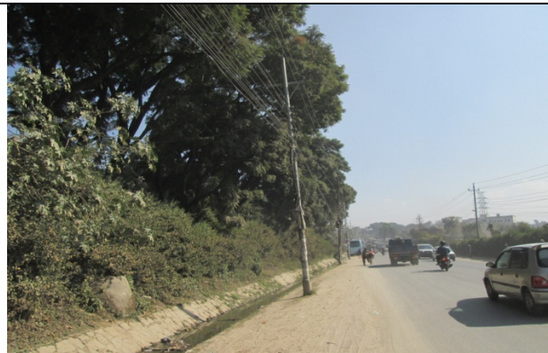
Figure 51. Surface storm water drain along road
