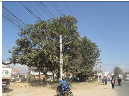
Figure 35. Electric pole no. 20
