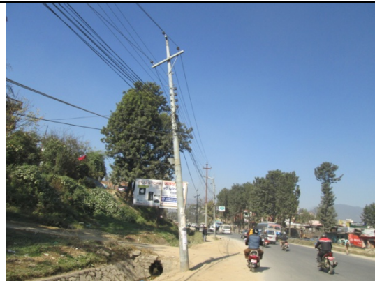
Figure 102. Electric pole no. 100
