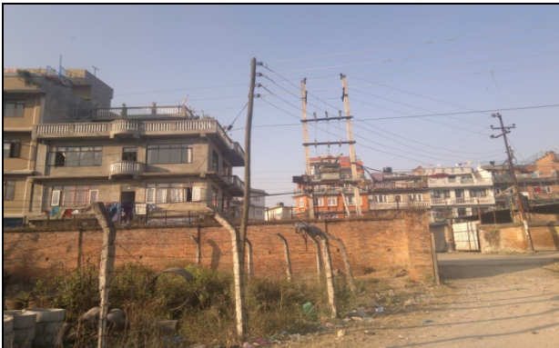
Figure 19. Electric pole no. 1
