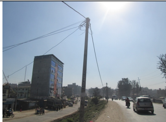
Figure 56. Electric pole no. 45
