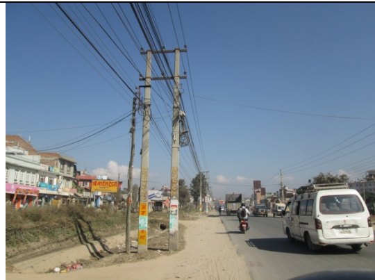
Figure 27. Electric pole no. 12
