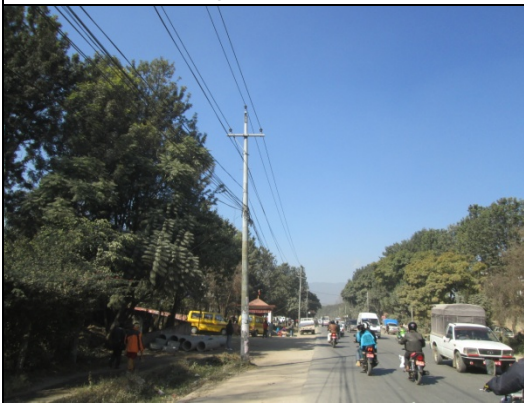
Figure 115. Electric pole no. 113
