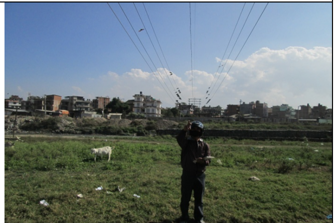
Figure 4. Transmission line passing across the site
