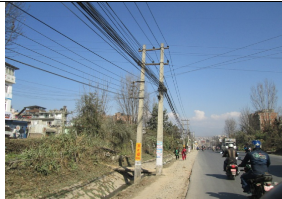
Figure 27. Electric pole no. 17
