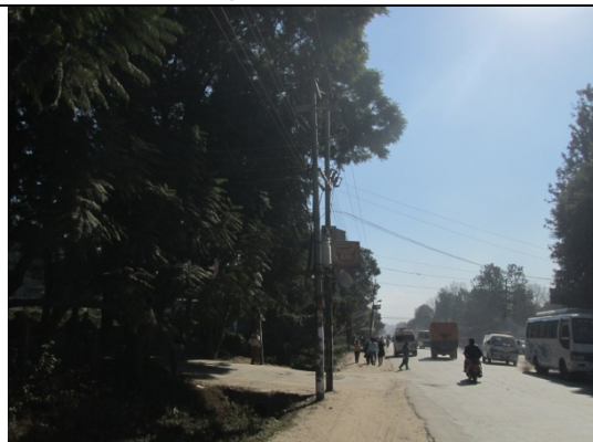
Figure 34. Electric pole no. 21
