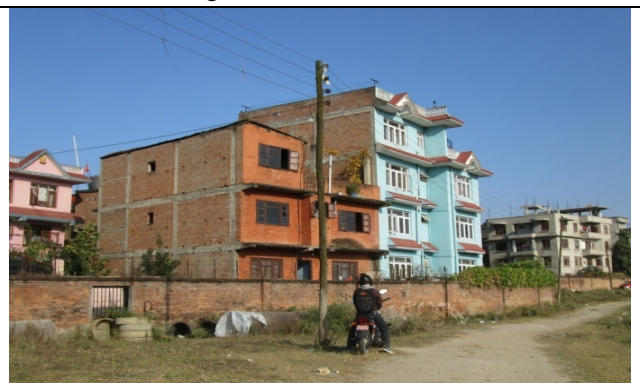
Figure 1. Electric pole no. 4
