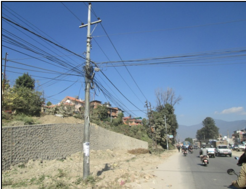
Figure 95. Electric pole no. 93
