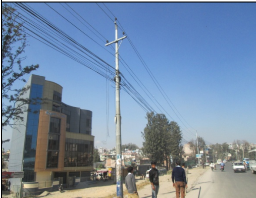
Figure 85. Electric pole no. 83
