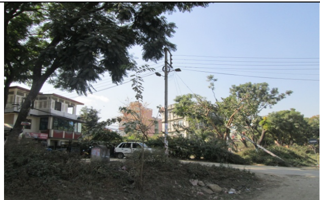
Figure 32. Electric pole no. 66
