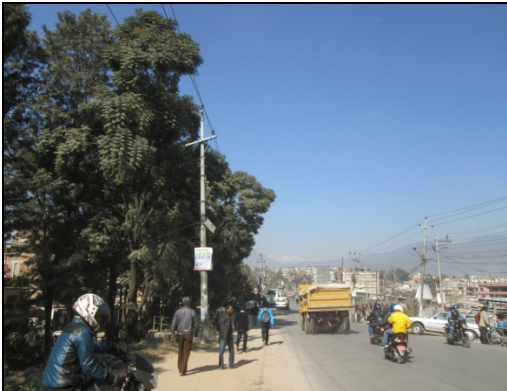
Figure 83. Electric poles no. 81
