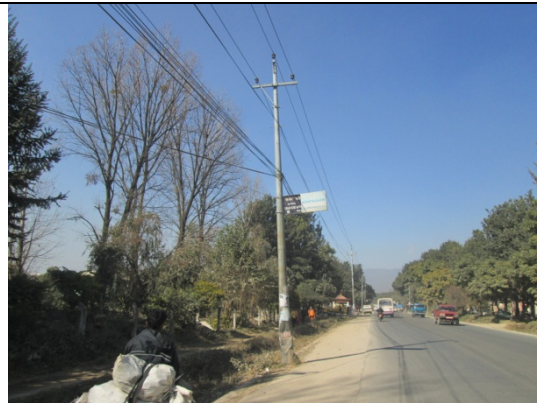
Figure 114. Electric pole no. 112
