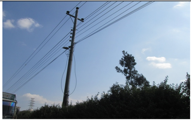
Figure 45. Electric pole no. 91
