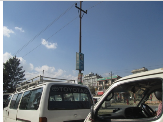
Figure 55. Electric pole no. 48
