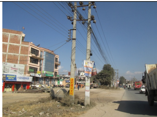
Figure 33. Electric pole no. 18
