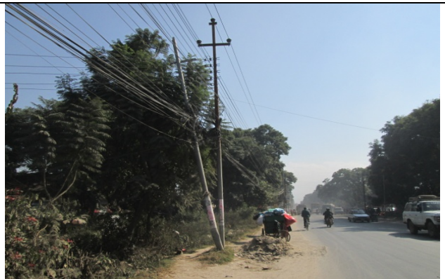
Figure 44. Electric pole no. 20
