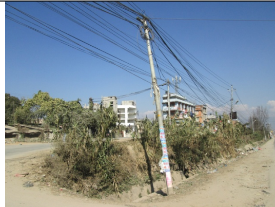
Figure 23. Electric pole no. 9
