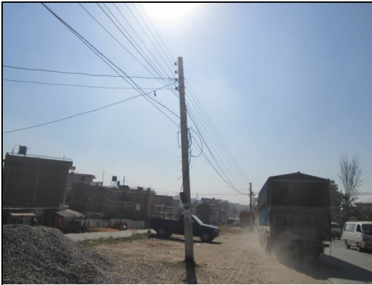
Figure 47. Electric pole no. 35
