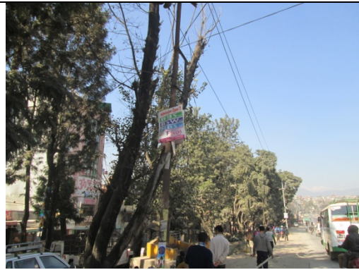
Figure 82. Electric pole no. 80
