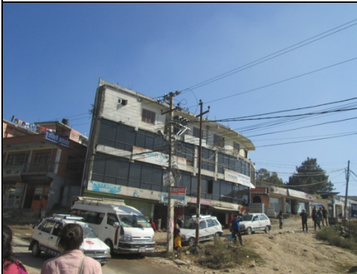
Figure 39. Electric poles no. 26 & 27
