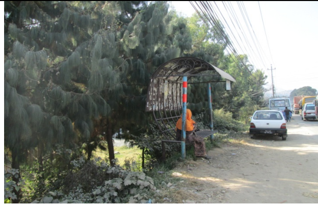
Figure 58. Temporary bus stand
