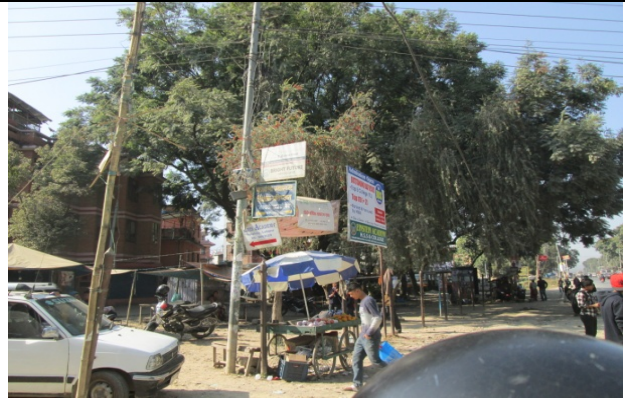
Figure 34. Electric pole no. 68
