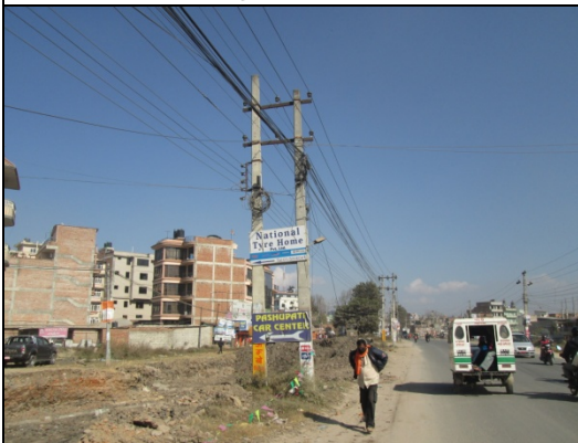
Figure 32. Electric pole no. 17
