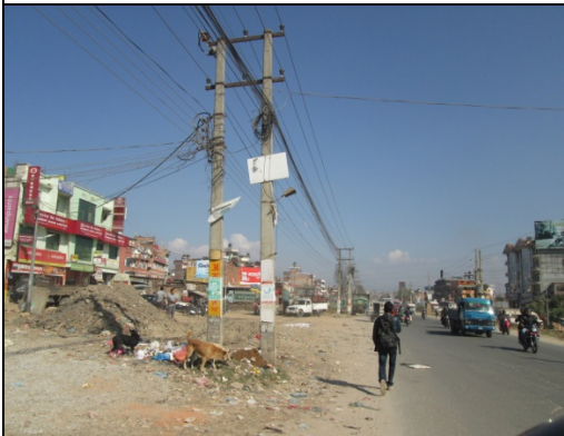
Figure 20. Electric pole no. 5
