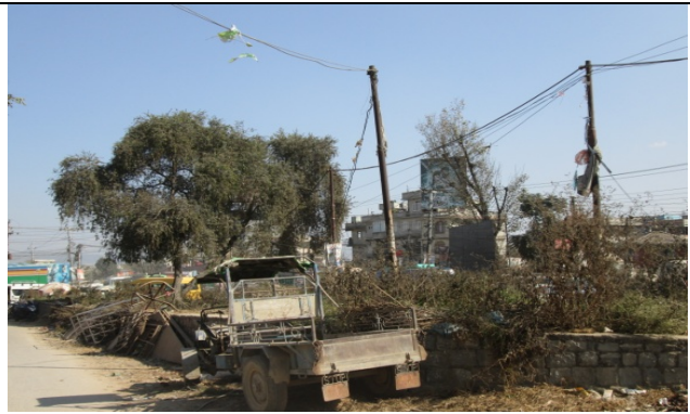
Figure 70. Electric pole no. 49 & 50
