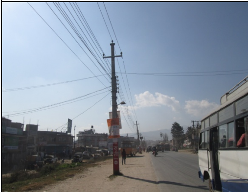
Figure 50. Electric pole no. 35
