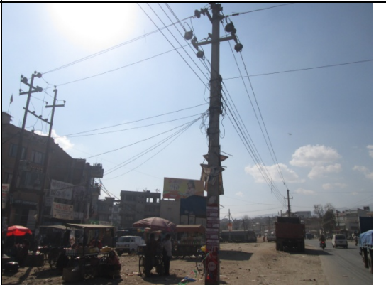
Figure 63. Electric pole no. 49
