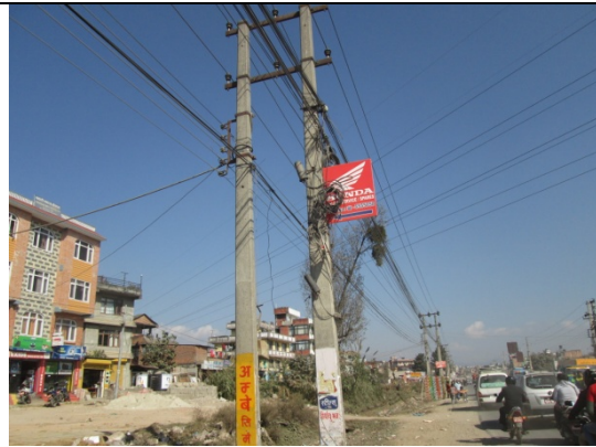
Figure 25. Electric pole no. 10
