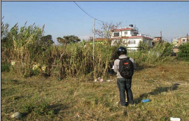
Figure 6. Electric pole no. 9
