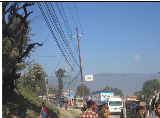
Figure 100. Electric pole no. 98
