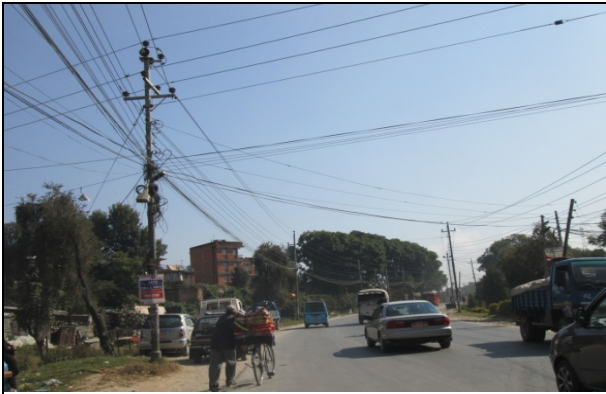
Figure 12. Electric pole no. 15
