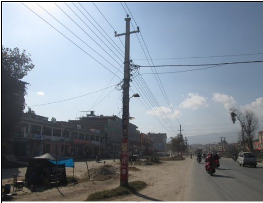
Figure 54. Electric pole no. 39
