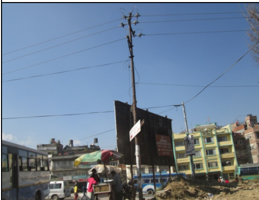
Figure 52. Electric pole no. 45
