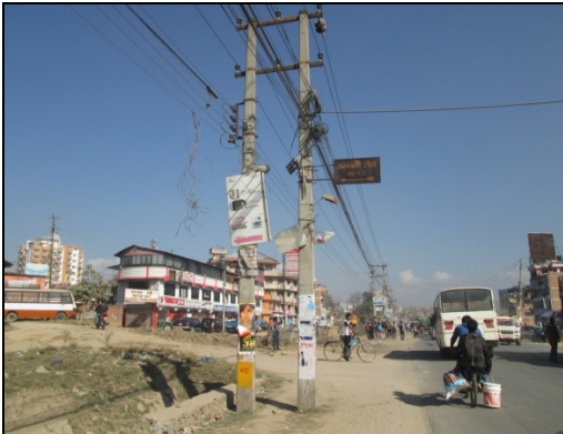
Figure 30. Electric pole no. 15
