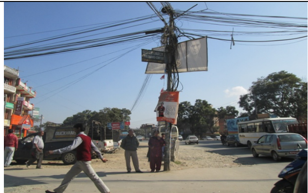
Figure 20. Electric pole no. 45
