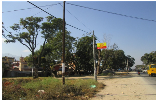
Figure 90. Electric pole no. 70
