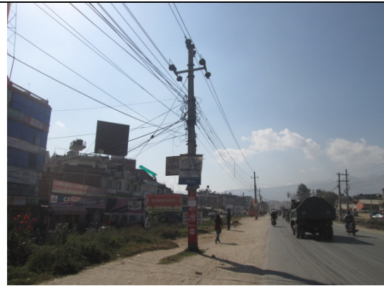
Figure 49. Electric pole no. 34
