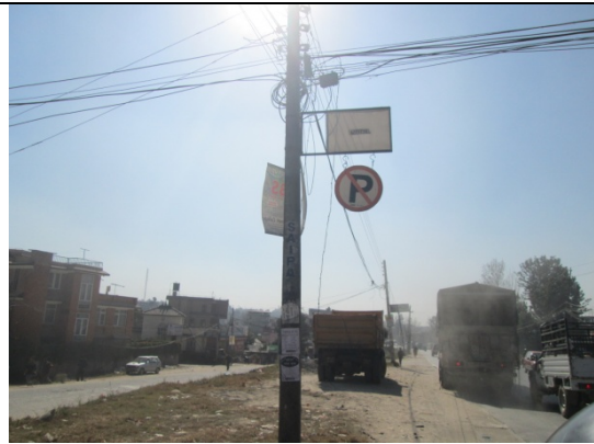
Figure 48. Electric pole no. 36
