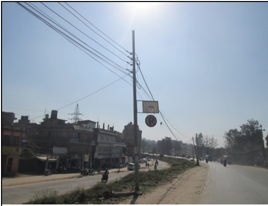
Figure 53. Electric pole no. 41
