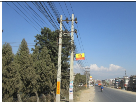
Figure 35. Electric pole no. 25
