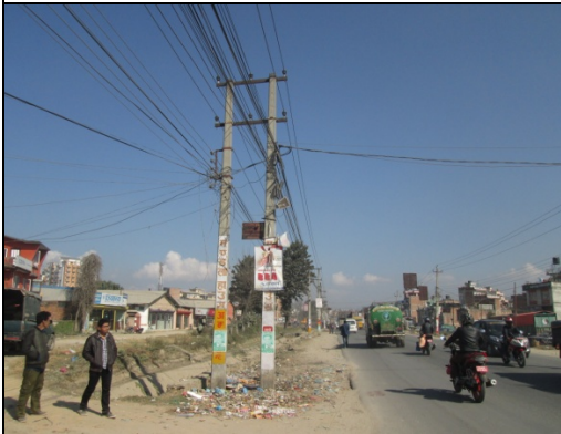
Figure 28. Electric pole no. 13
