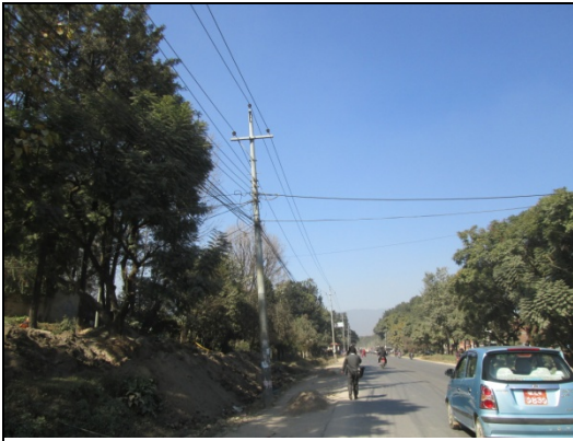
Figure 113. Electric pole no. 111
