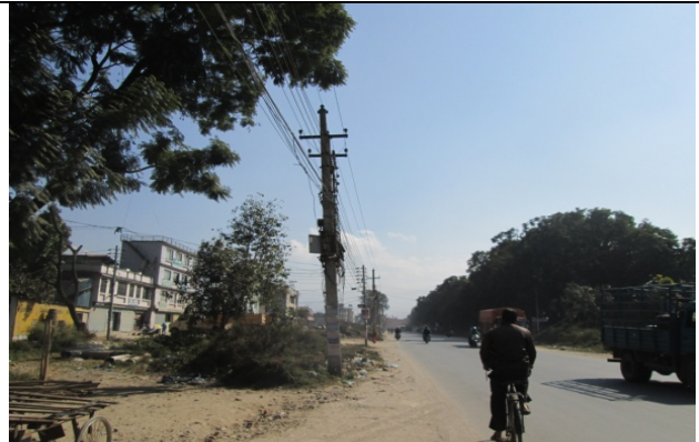
Figure 56. Electric pole no. 32
