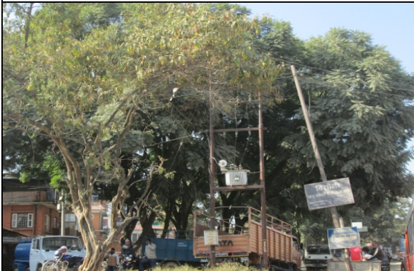
Figure 83. Electric pole no. 63
