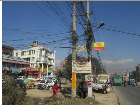
Figure 33. Electric pole no. 23
