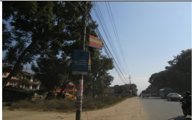
Figure 42. Electric pole no. 18
