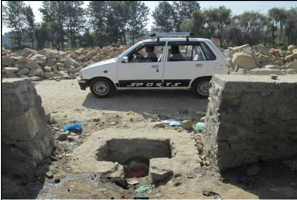
Figure 2. Inlet of underground sewer no. 3
