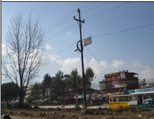
Figure 50. Electric pole no. 43
