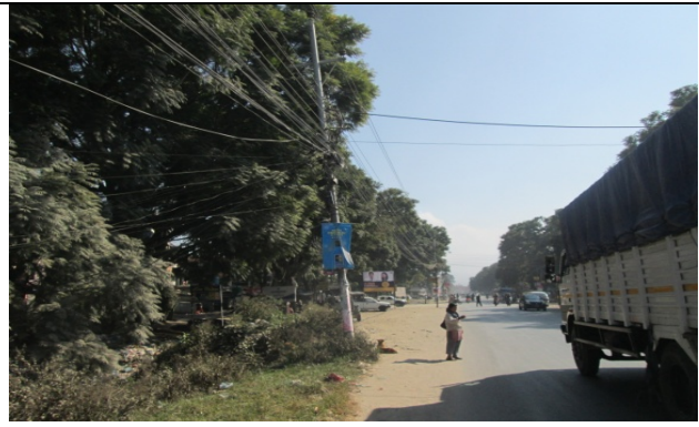
Figure 52. Electric pole no. 28
