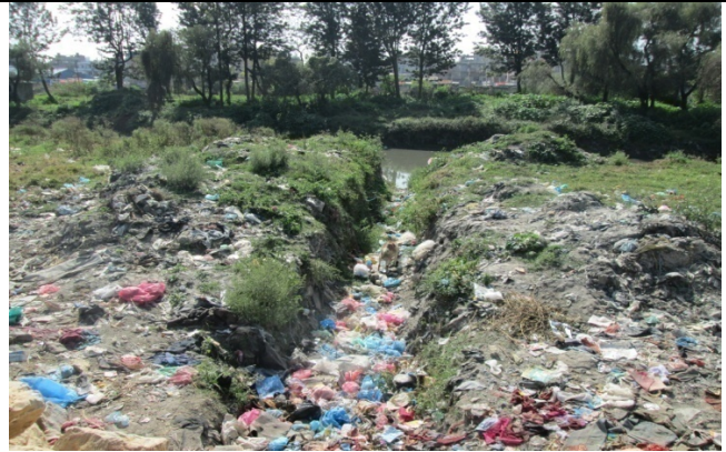
Figure 3. Outlet of incomplete underground sewer no. 3
