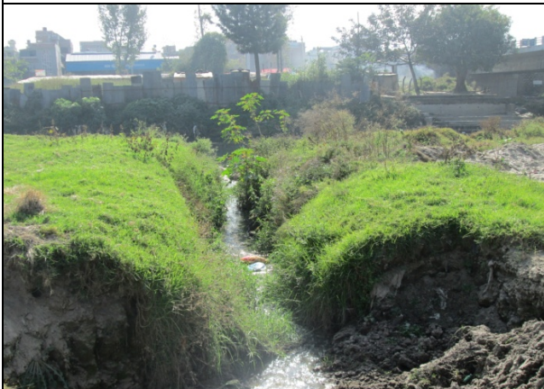
Figure 13. Inlet of Surface Storm water drainage no. 2 and sewer no. 2
