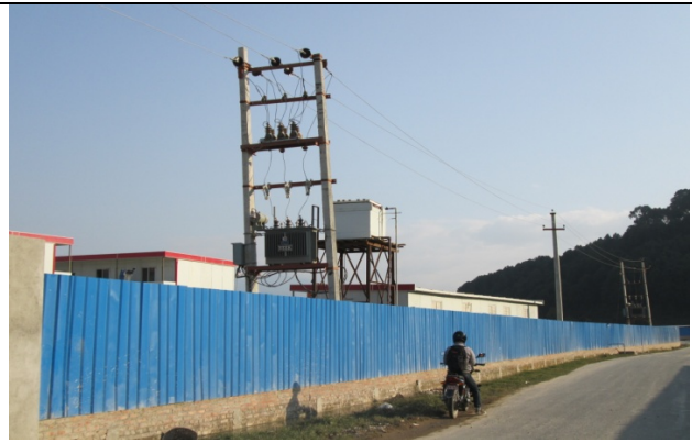
Figure 15. Electric pole no. 20
