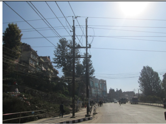
Figure 72. Electric pole no. 68
