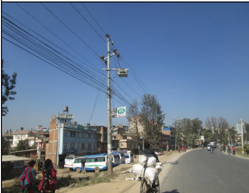
Figure 87. Electric pole no. 85
