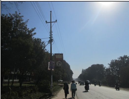
Figure 31. Electric pole no. 18
