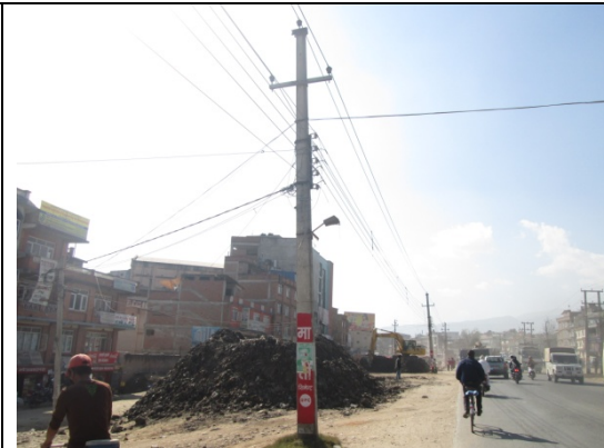
Figure 61. Electric pole no. 47
