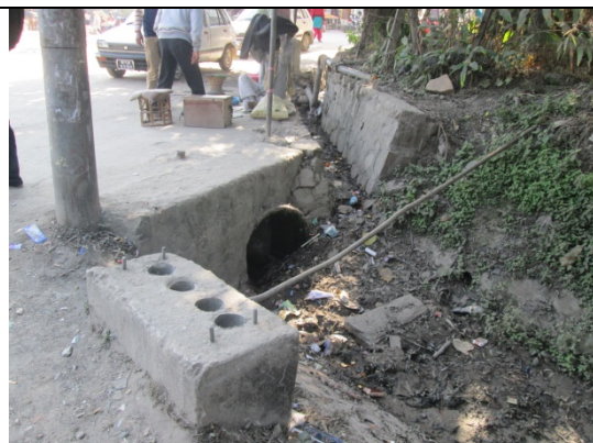
Figure 128. Surface storm water drain along road
