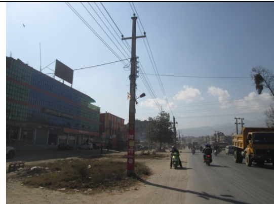
Figure 55. Electric pole no. 40
