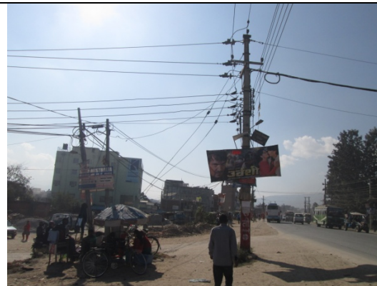
Figure 45. Electric pole no. 30
