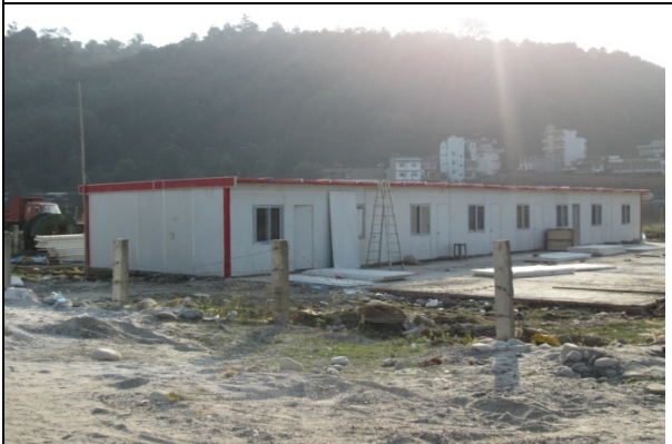
Figure 51. Office Building of Chinese ring road expansion team ( no. 7)
