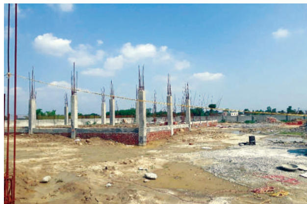
Construction of Civil Structure
