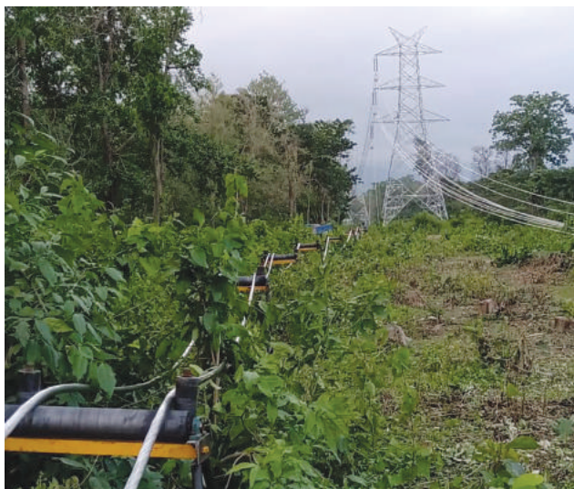
Stringing work undergoing in plain section
