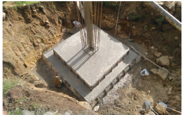
Tower foundation under construction
