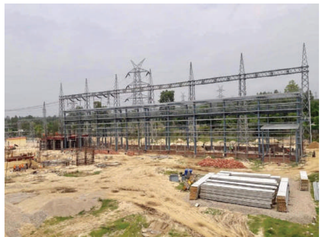
Under construction 400 kV GIS Substation at Dhalkebar
