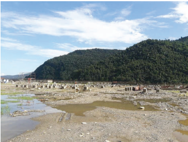
Lahachowk Switchyard Foundation
