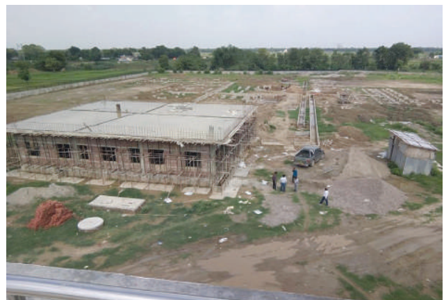
Mainahiya S/S Civil Works Progress
