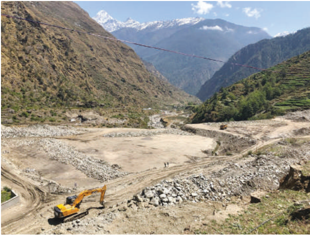
Chilime Hub Substation Site after completion of cutting filling and compaction
