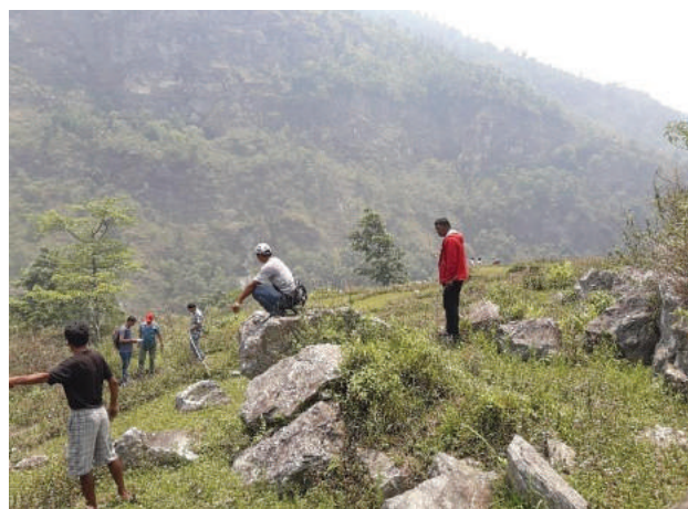
Survey works at Rahughat Substation
