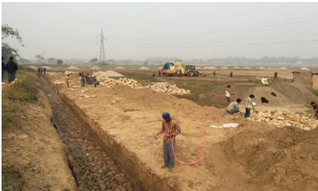
Construction of Boundary Wall
