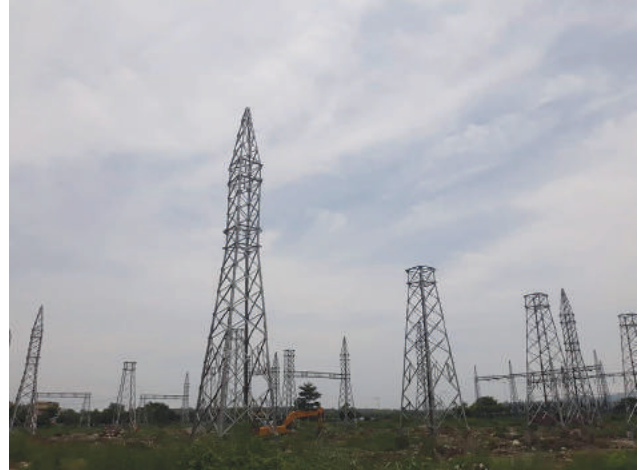
Erected Gantry Towers at 220/132 kV Hetauda Substation
