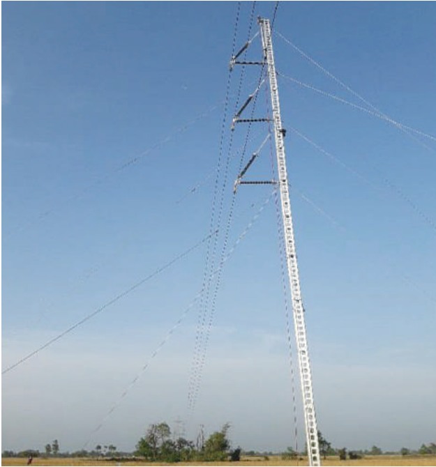
ERS Tower After Completion
