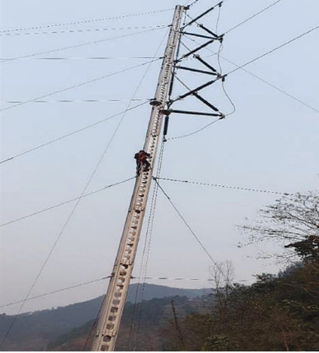
ERS Tower just after Completion
