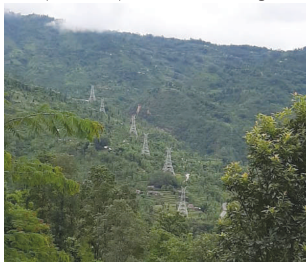
Tower erection ongoing
