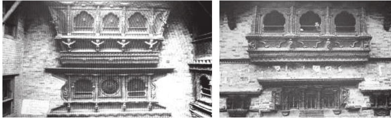
Sa: Jhaya (Three Bay Window)
