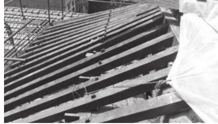
Layout of Rafters at Roof
