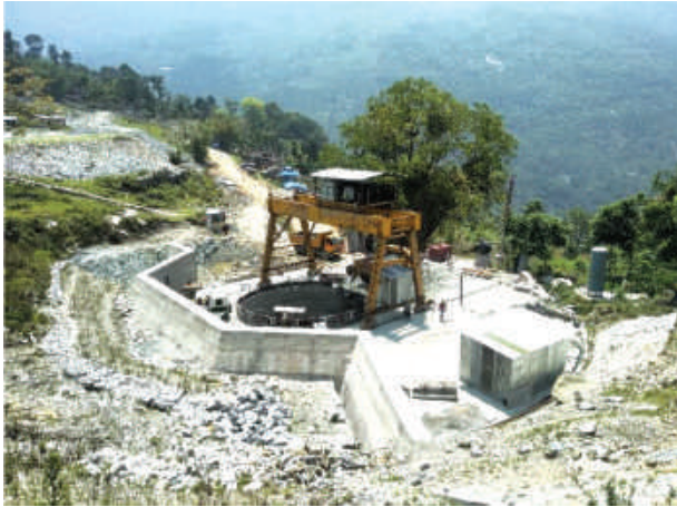
Work in Progress in Surge Shaft
