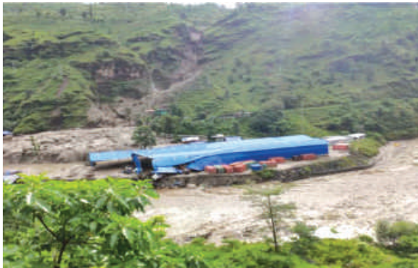
Flood impact on Storage yard of Lot-2 (Electromechanical works)
