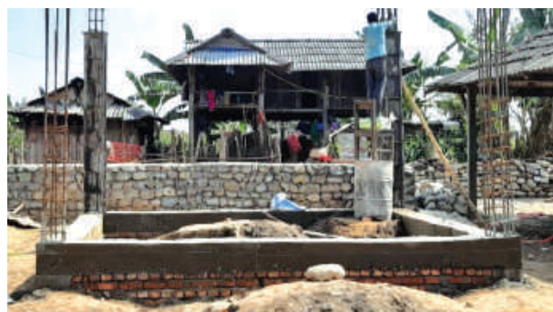
Under construction School Office Room in Nijgadh, Bara
