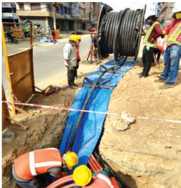
Cable laying works at Chabahil
