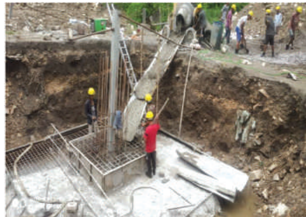
Tower Foundation work in progress: Udipur-Bharatpur 220 kV Transmission Line
