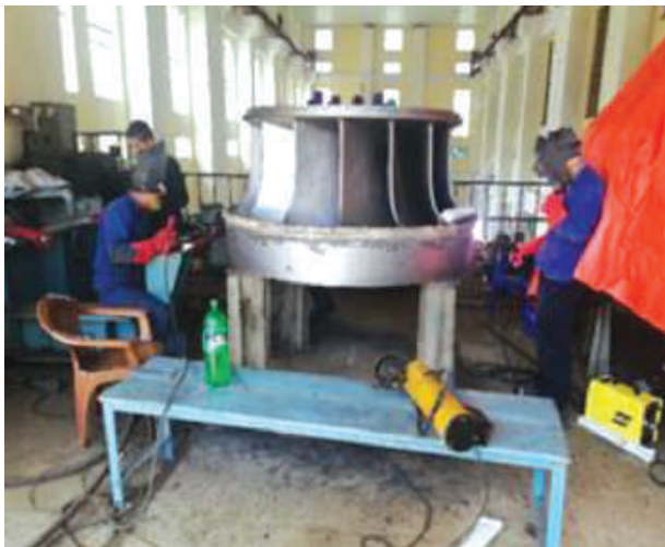
Welding of Francis Runner
