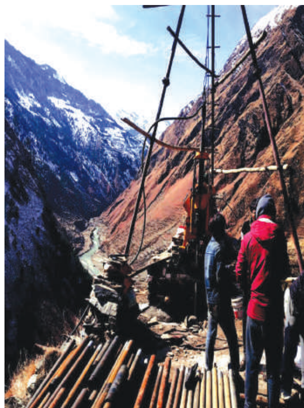
Drilling work at JSHEP
