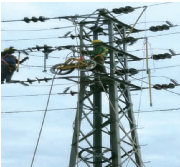
ACSR Conductor Replacing by ACCC conductor in Dhalkebar Mujeliya 33 kV Line
