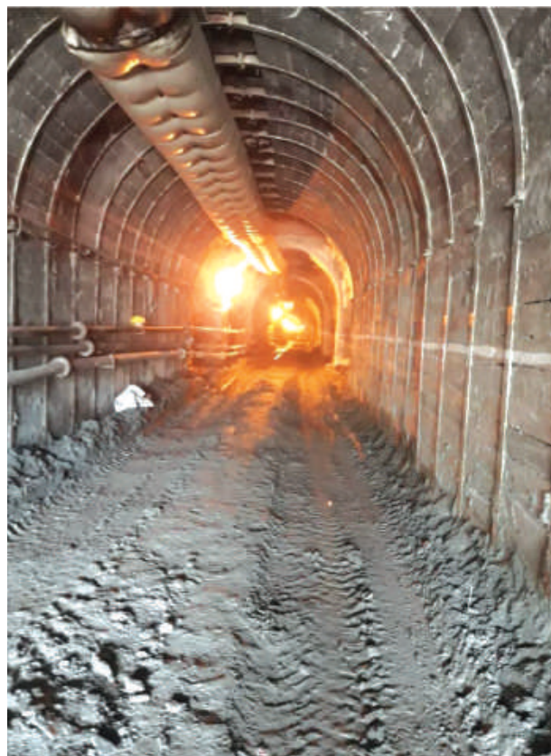
Work in Progress in Adit-3
