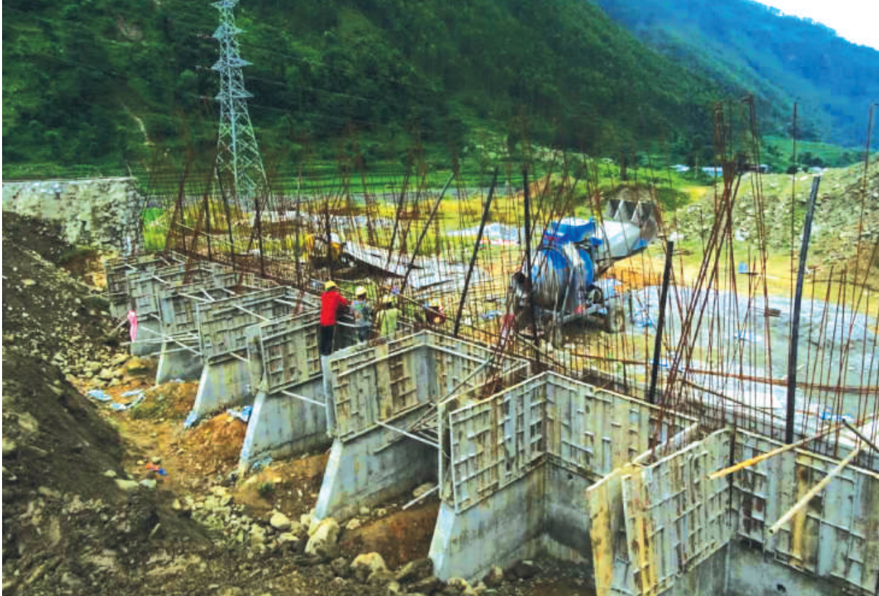
Under-constructing Trishuli 3B Hub Substation
