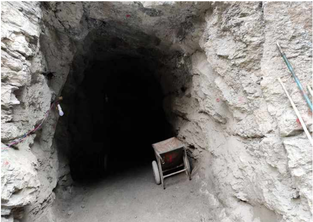
Test Adit at Proposed Headworks Site
