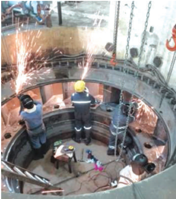
Repairing of Stay vanes
