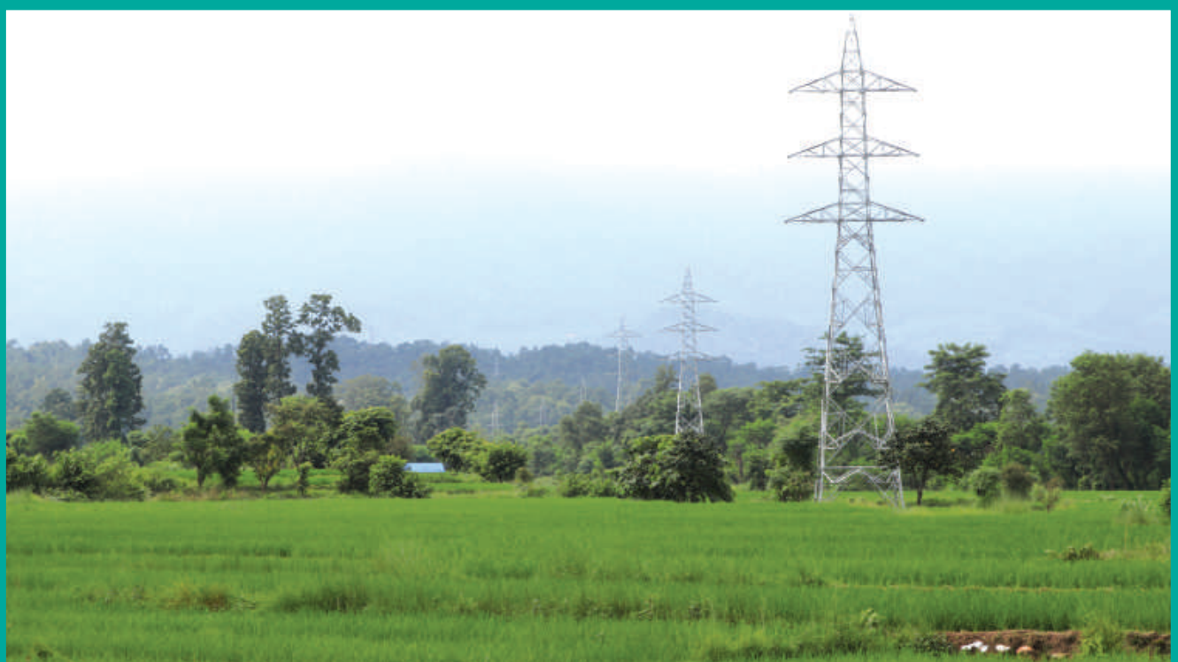
Bardaghat – Sardi 132 kV Transmission Line Tower Erection
