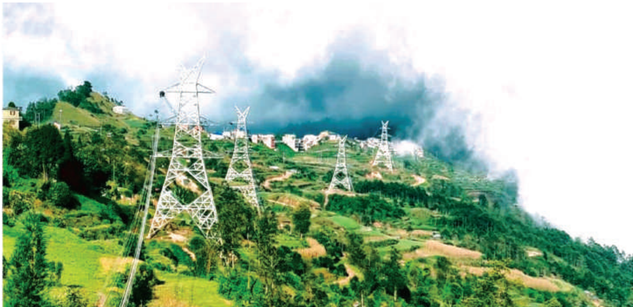
Ongoing Stringing work at Dhankuta Section
