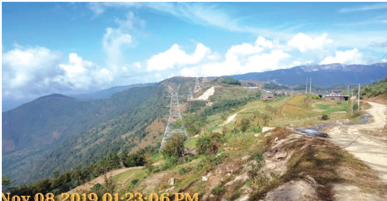
Stringing work under progress at Chitre, Dhankuta District.
