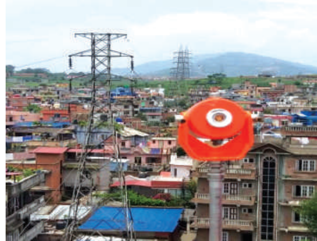
Detail Survey of Patan Suichatar 66 kV Transmission Line, Houses constructed in RoW
