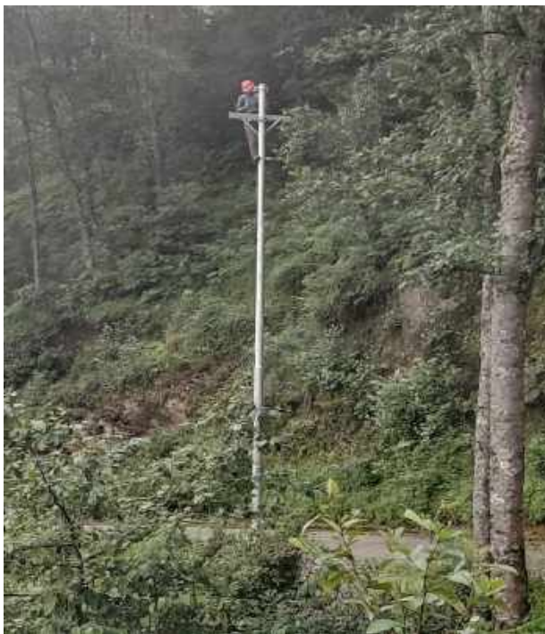
Installation of hardware for poles at Solukhumbu District
