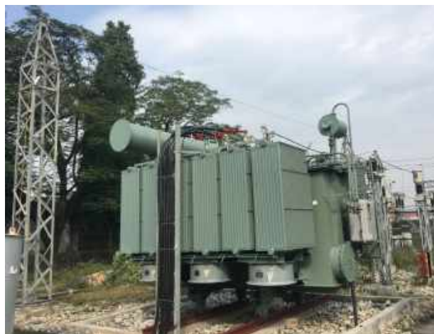
Substation Upgradation at Mahendranagar DC, Kanchanpur
