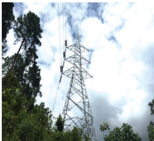
Conductor Stringing in one circuit in 132 kV Tower
