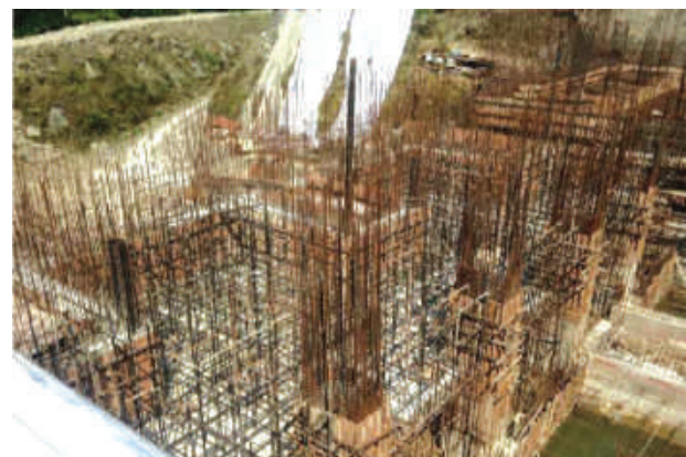
Reinforcement placement in Powerhouse
