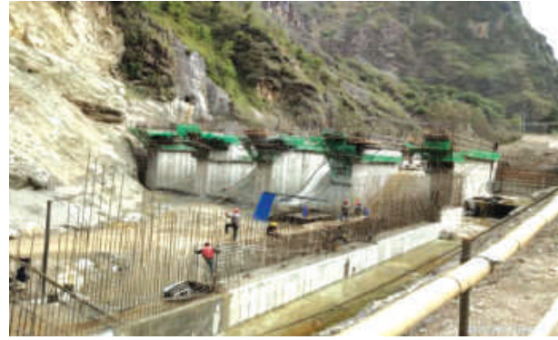
Construction of Dam in progress
