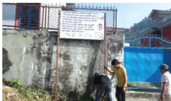
Hoarding Board Installation at Bhalamchaur, Pokhara Metropolitan City
