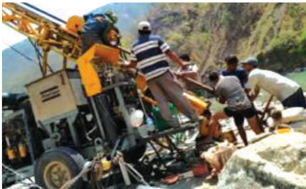
Core Drilling Works at Dudhkoshi SHEP.
