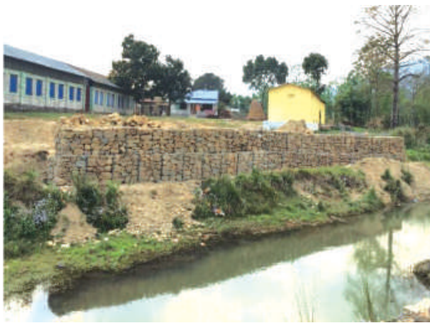
River bank protection at Gaidakot, Nawalpur
