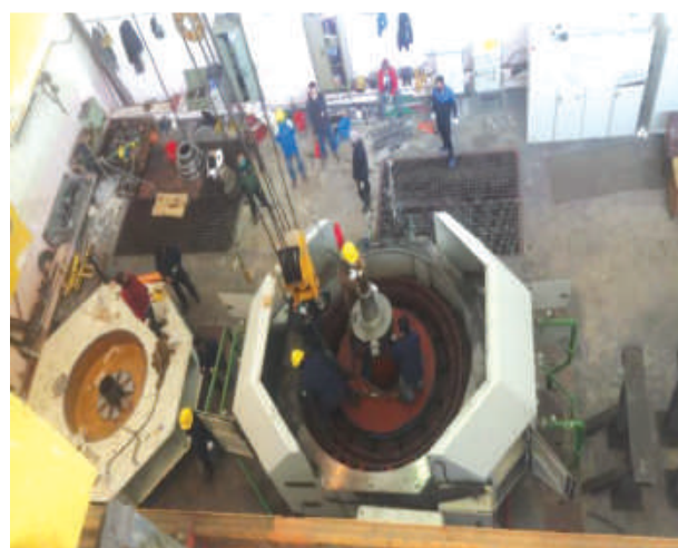
Installation of Rotor Shaft during overhauling
