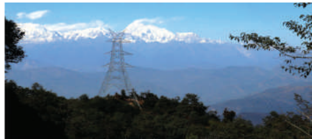
Tower Erection under progress in Basantapur-Dhungesanghu section
