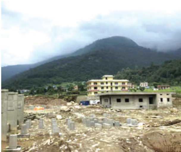
Under construction Garjyang substation
