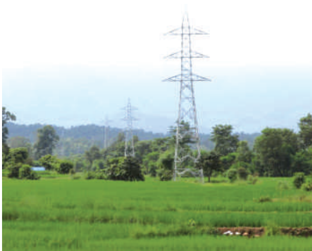
132 kV Tower Erection at Sardi
