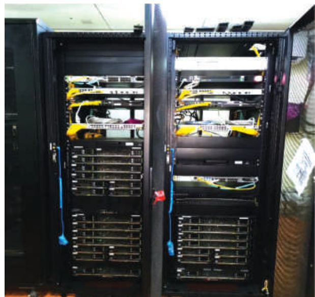
Data Centre construction at IT Department premises
