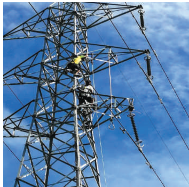
Cross Arm Maintenance works
