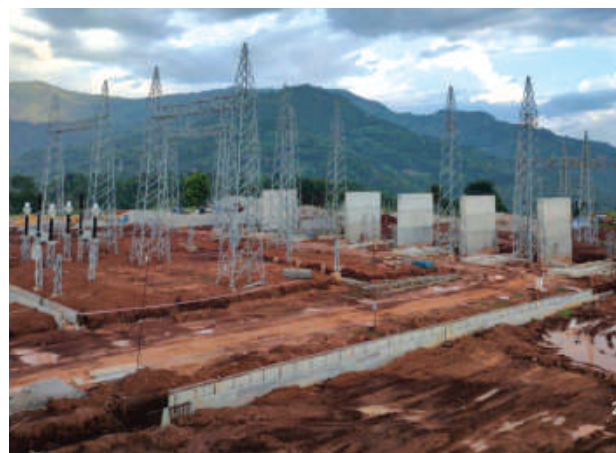
Constructional activities at Tumlingtar Substation
