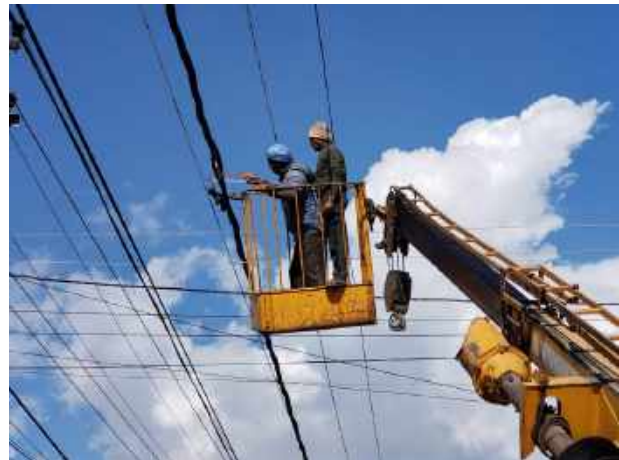
Tatopani Feeder maintenance work after Burnt Suska Cable at Pokhara DC
