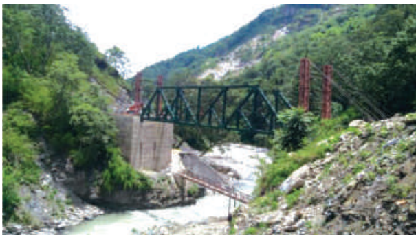
Work in Progress in Permanent Bridge
