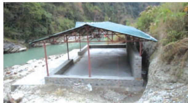
Construction of Shade at Phulbari Ghat, Sundarbazar, Lamjung
