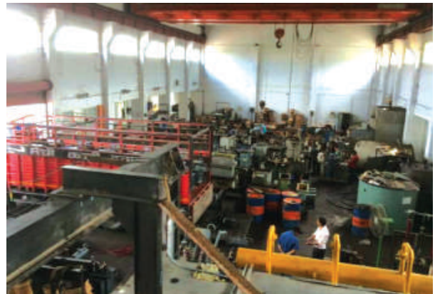
Inside Transformer Workshop
