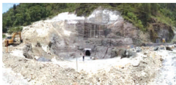
Work in Progress in Power House
