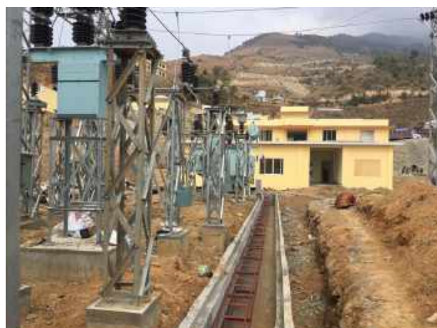
Construction of Cable Trench for cabling works during substation construction
