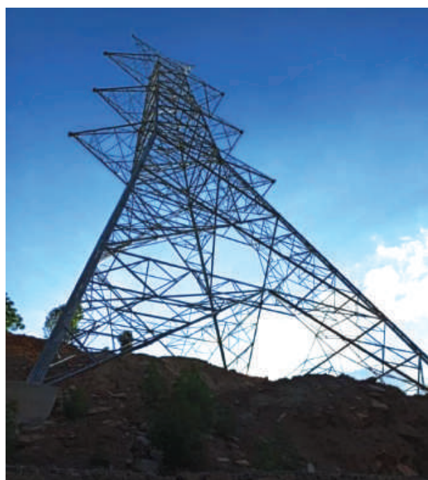
400 kV Bahrabise-Kathmandu Transmission Line Tower
