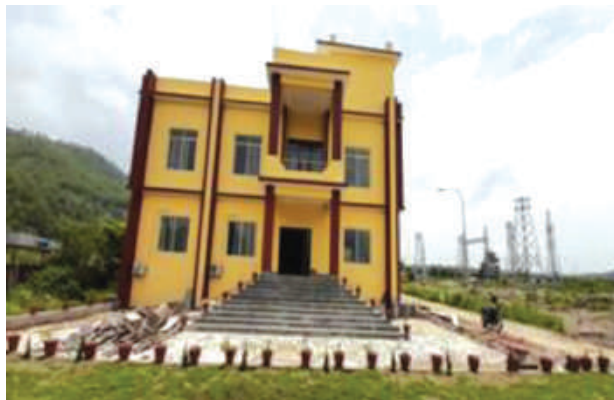
Emergency Control Center (ECC) Building at Hetauda
