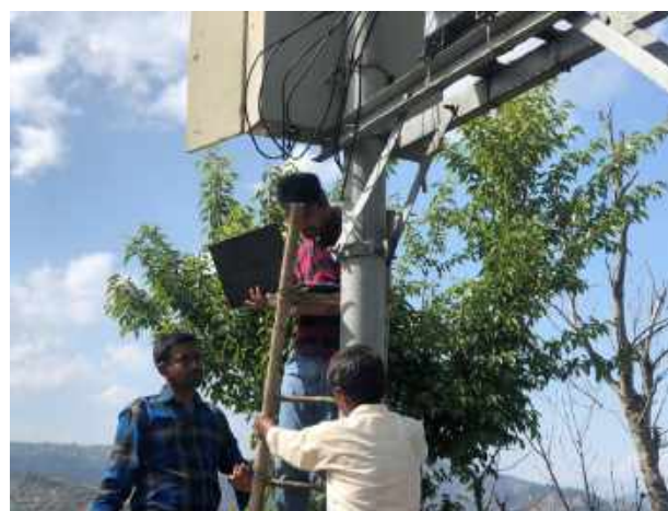
Installation and configuration of AMR modem in TOD Meter
