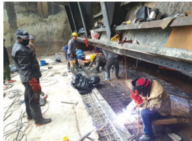
Replacement of sill plate of gate no. 3 of diversion weir
