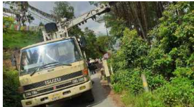
Bush Cutting activities under Kuleshor Distribution Center
