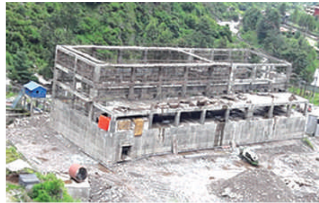
HEP Headworks & Powerhouse
