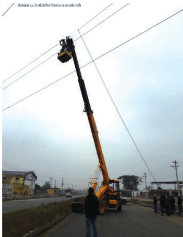
Repairing work of broken strands of conductor near Simara
