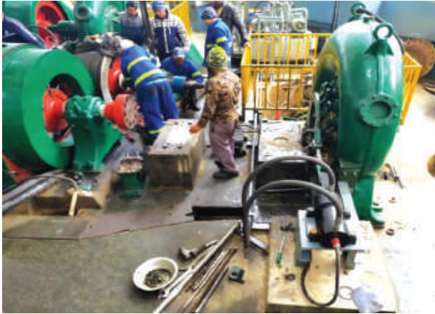
Turbine Overhauling of unit no. 3
