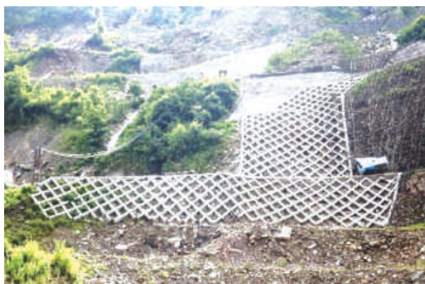
Powerhouse Slope Support
