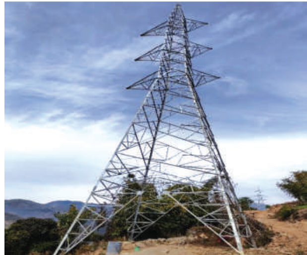
132 kV Transmission Tower
