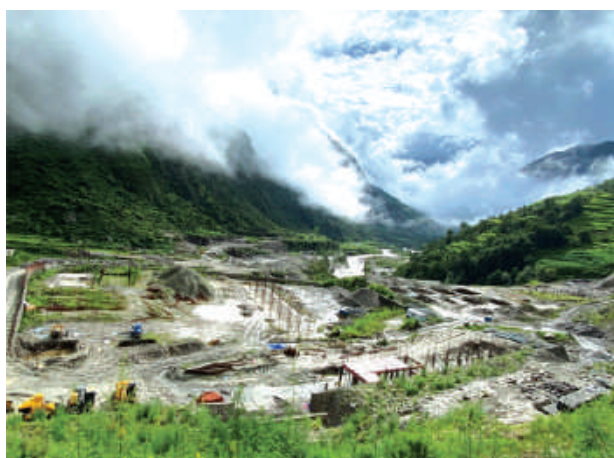
Chillime Hub substation site, various construction activities are ongoing.
