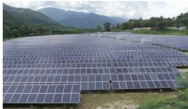
Solar Farm under construction at Devighat
