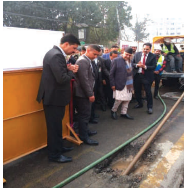
Horizontal drilling for Distribution system undergrounding in Maharajgunj area
