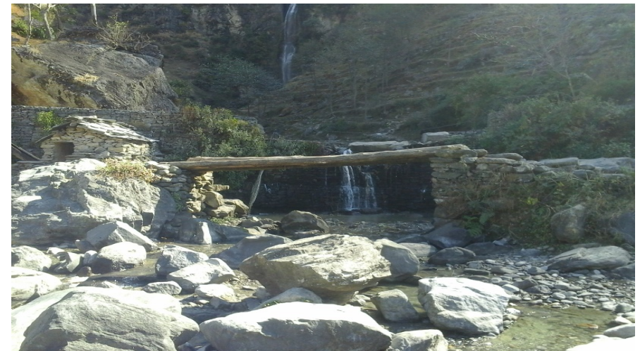
Caption:Elevation view from downstream
