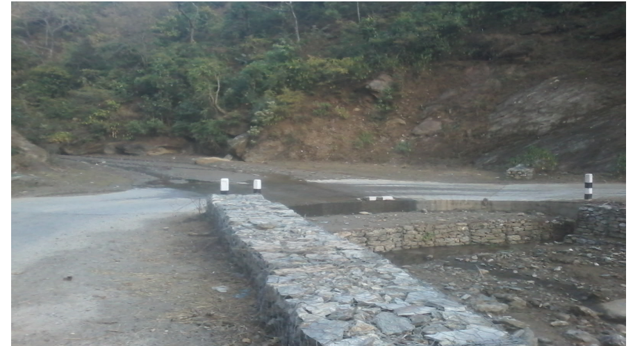
Caption:bridge site (existing facility is causeway)
