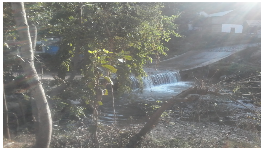
Caption:Existing vented causeway
