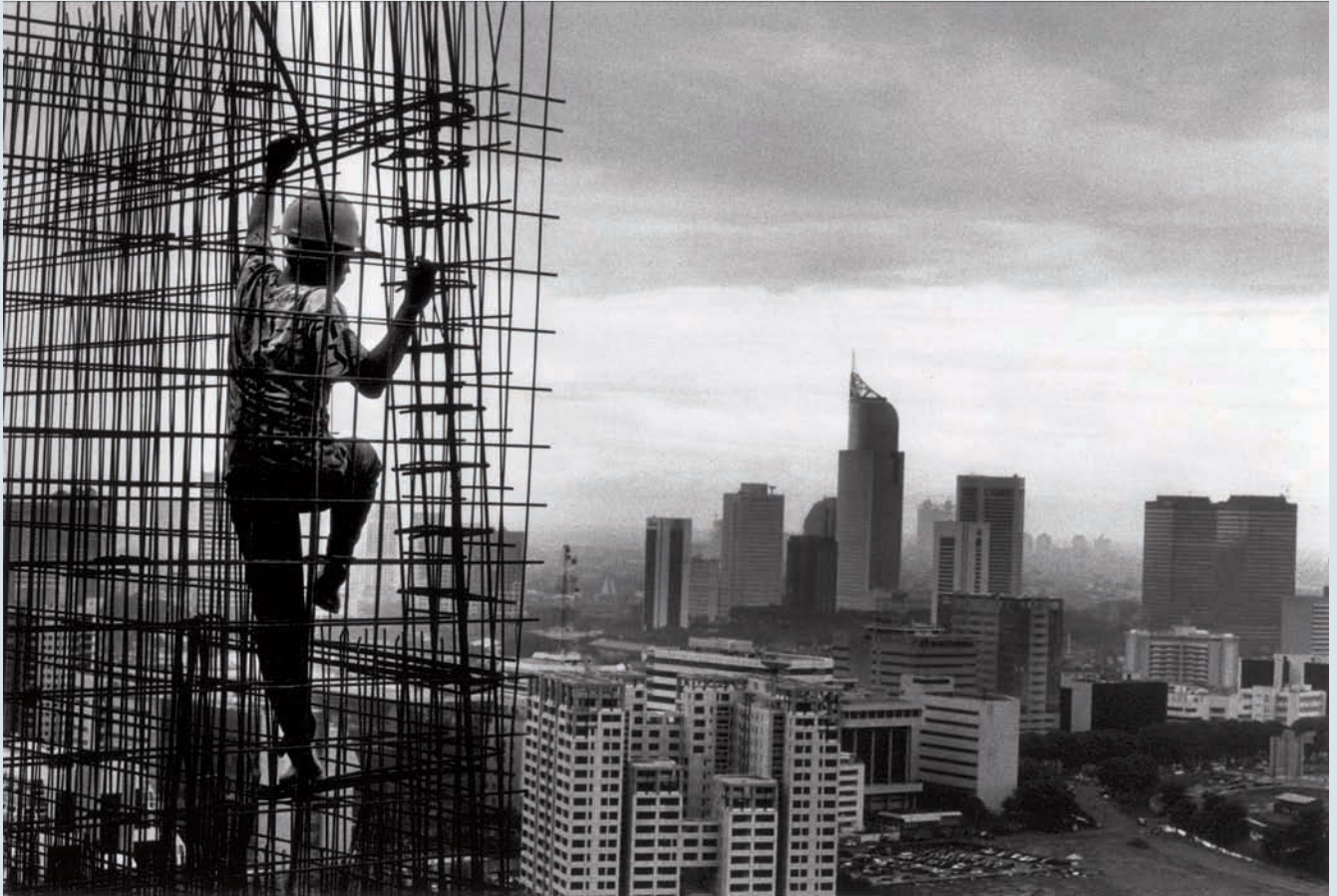
Worker at a construction site in Jakarta, Indonesia
