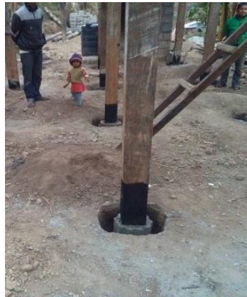
Excavate the soil around the column and construct stone/brick masonry.
