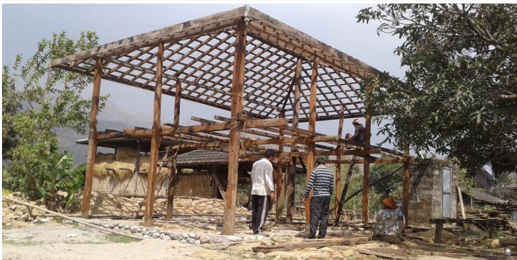
Figure is shown in traditional of timber framed structures in Siwalik range.
