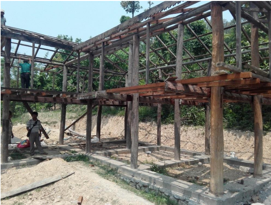
RCC Plinth band
