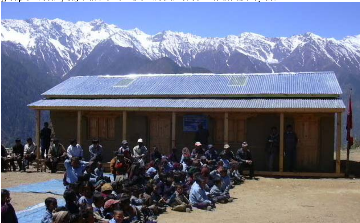
Plate 8. School building built by one of the women groups in Humla.
