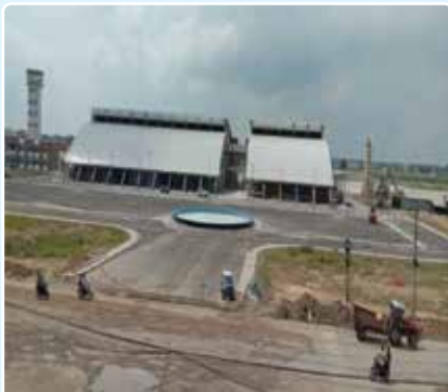
View of Control tower and ITB
