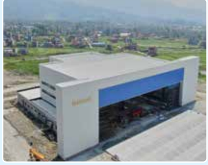
Arial View Hangar Building
